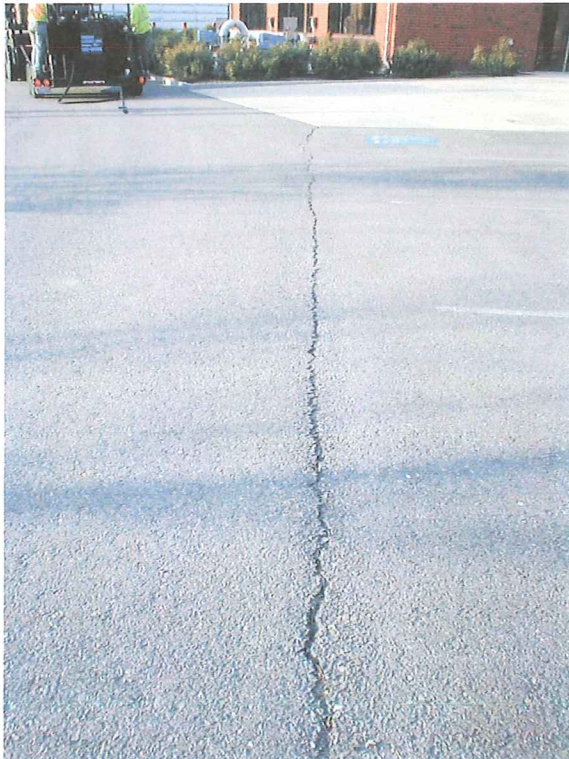
The WWTF driveway underwent crack repair on April 10 th – above are typical before and after pictures.
