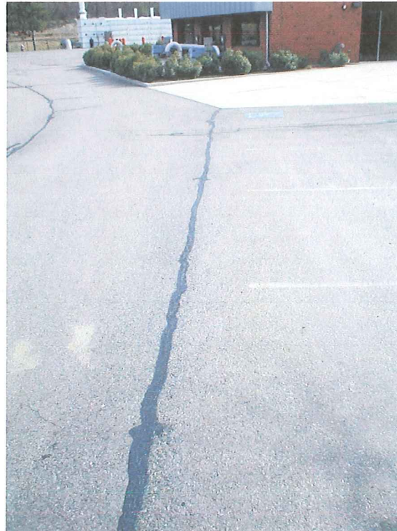
The WWTF driveway underwent crack repair on April 10 th – above are typical before and after pictures.
