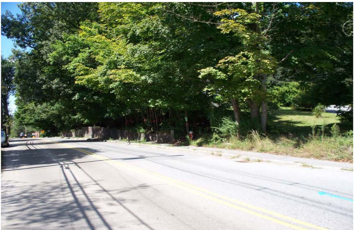
Route 62 Retaining Wall Near Damon Mill – Trees on Right will be removed to construct new stone wall. New trees will replace existing.
