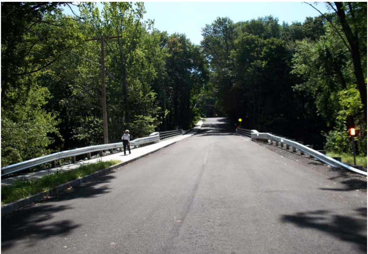
New Pine Street Bridge now open to all traffic (looking east toward Upland Road)
