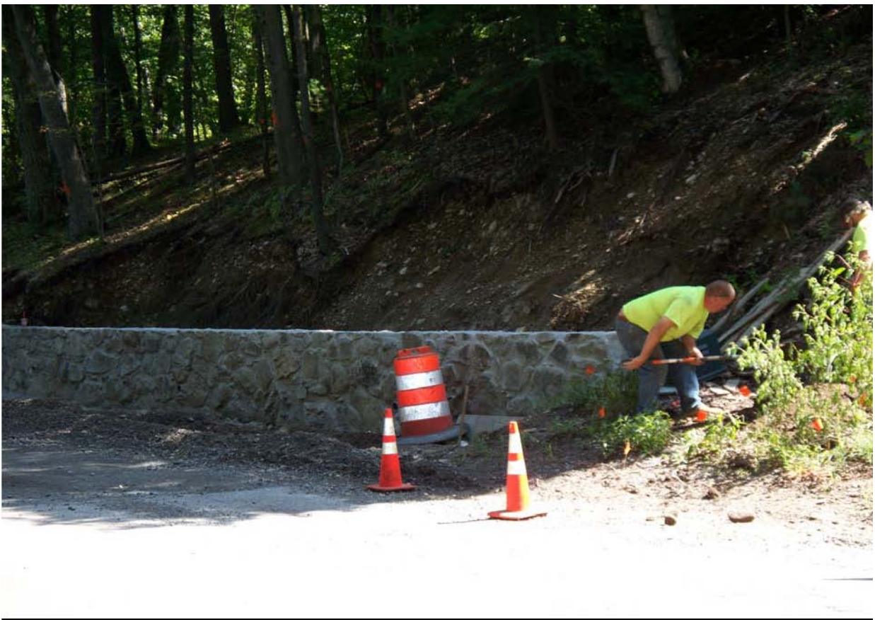
New Retaining on Main Street (Rt 62) North Side
