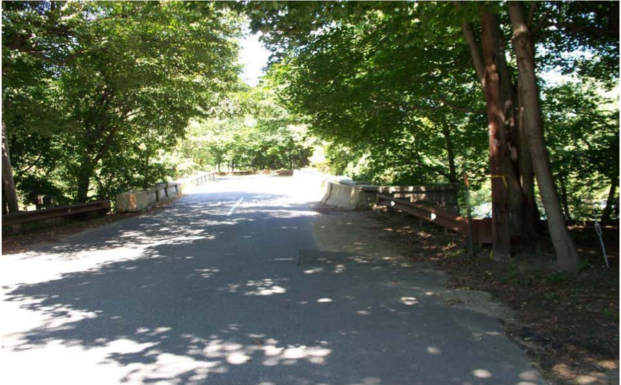
Nashawtuc Bridge will be closed for repairs September 1 through November 30.
