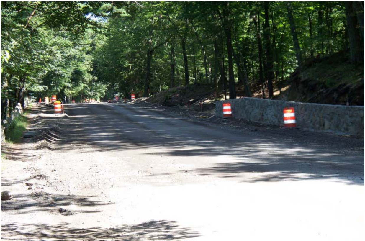
Work Continuing on Main Street (Route 62) – Paving to begin Sept 3
