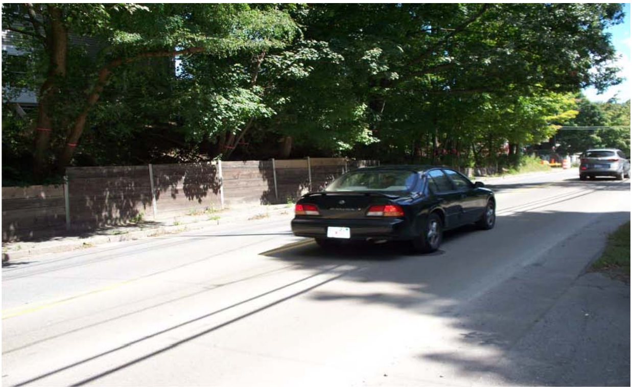
New Stone Retaining Wall will replace existing wall on Rt 62 near Damon Mill
