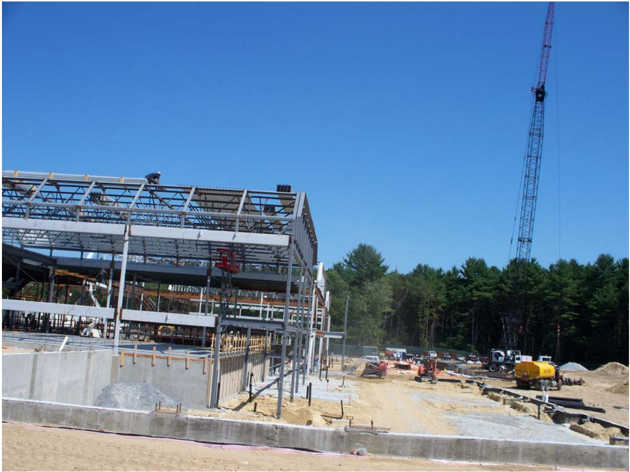
Steel Erection Progressing at New Willard School
