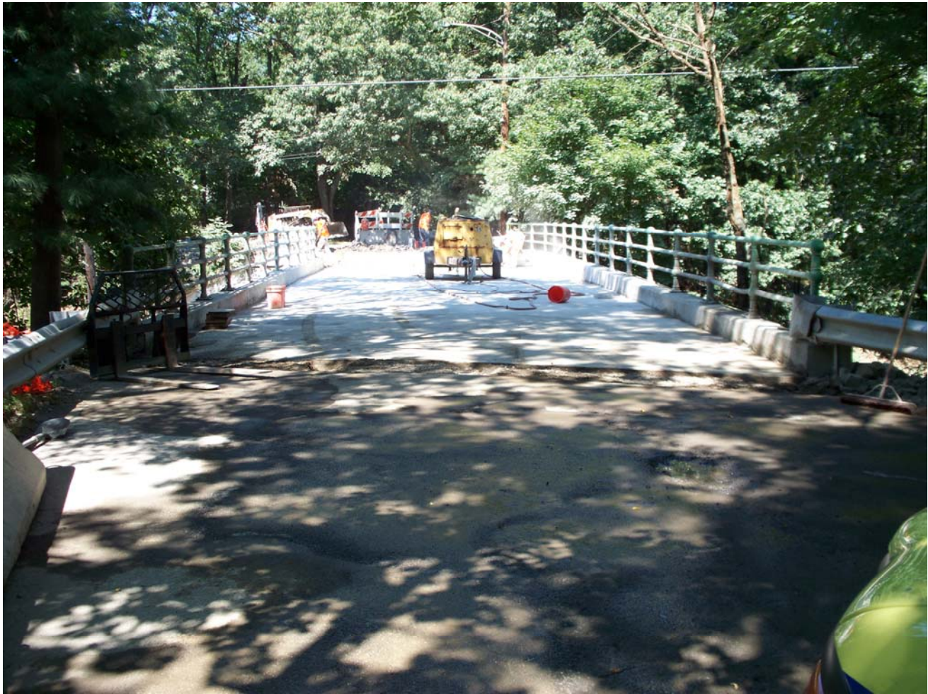
Concrete Deck Has Been Poured on Old Stow Road Bridge
