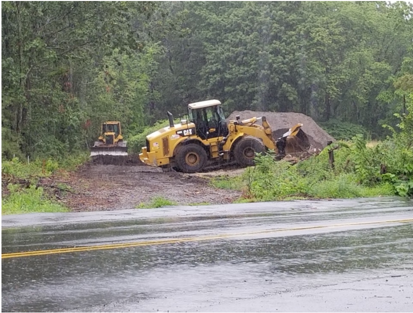
EARTHWORK AT THE NORTHERN MOST PORTION.
