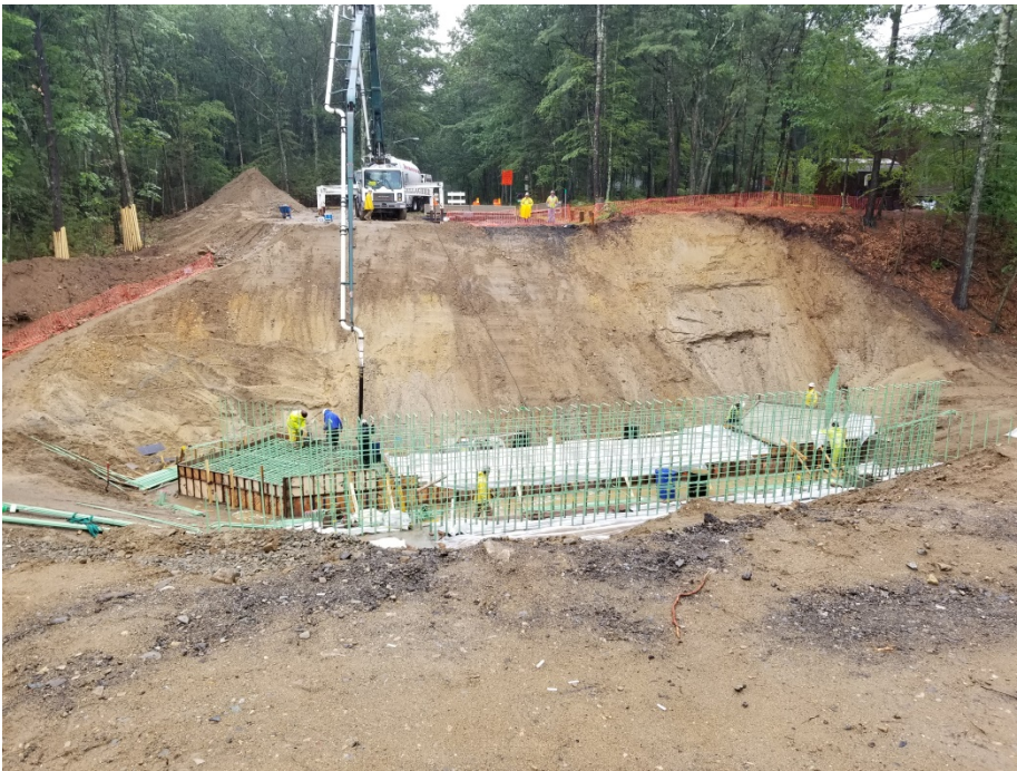
CONCRETE PUMPED FROM POWDER MILL ROAD
