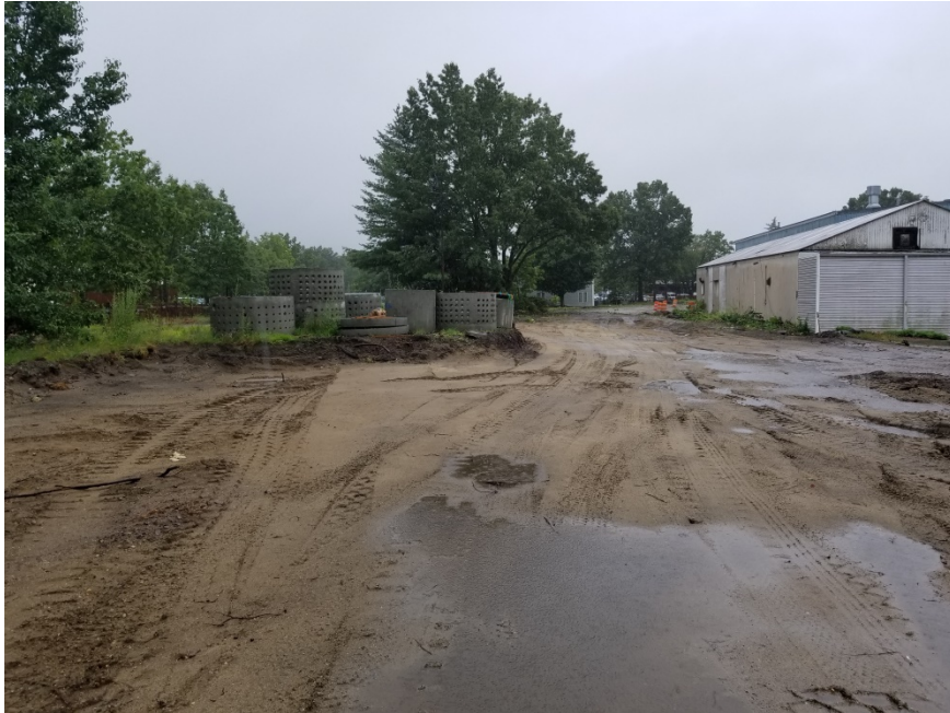
LEACHING CATCH BASINS AWAITING INSTALLATION
