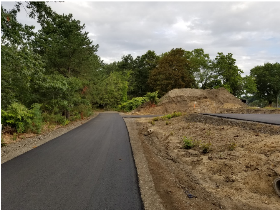
NORTHERN END OF THE PROJECT
