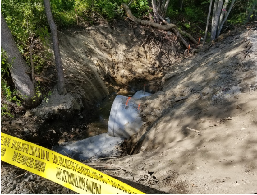
CULVERT INSTALLED AT STATION 81+10
