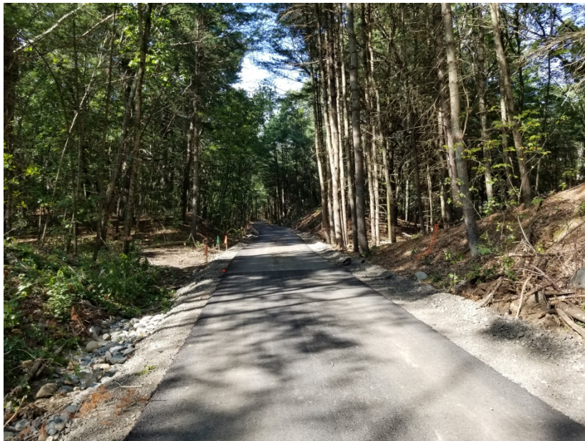
PORTIONS OF THE PROJECT ARE PAVED
