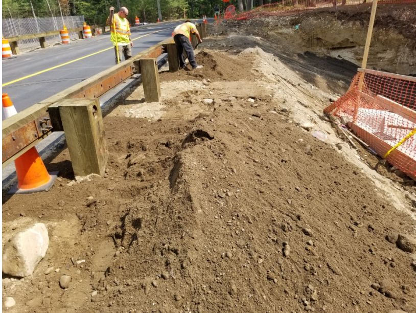
FINAL GRADING OF SIDESLOPES AT POWDER MILL ROAD
