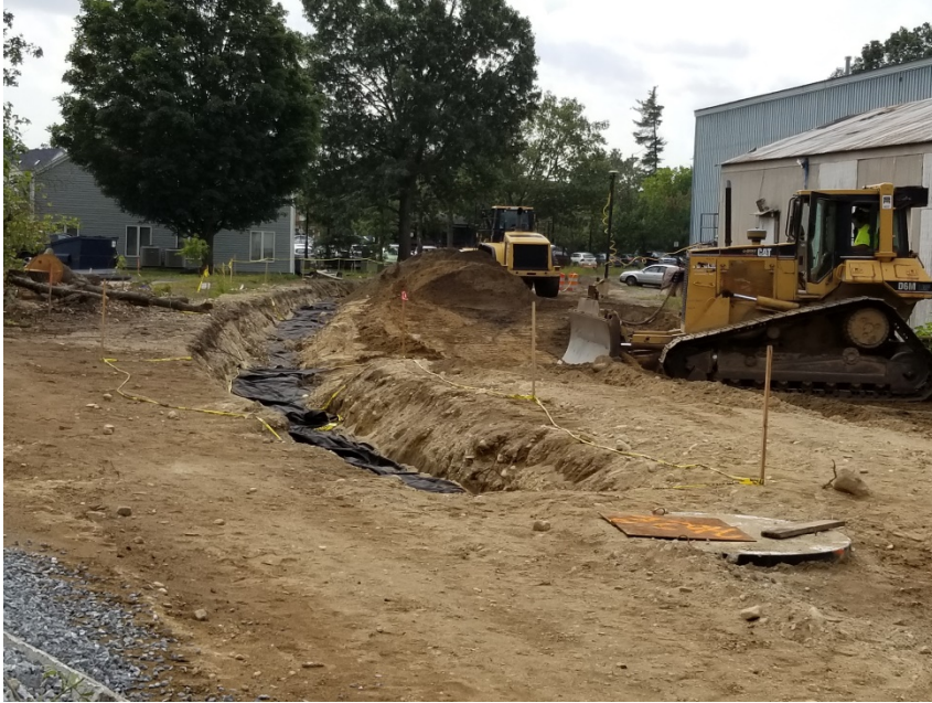
EARTHWORK IN THE VICINITY OF BROOKSIDE SQUARE FOR UTILITY INSTALLATION
