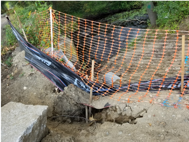
EDGE OF WORK AREA WITH EROSION CONTROL
