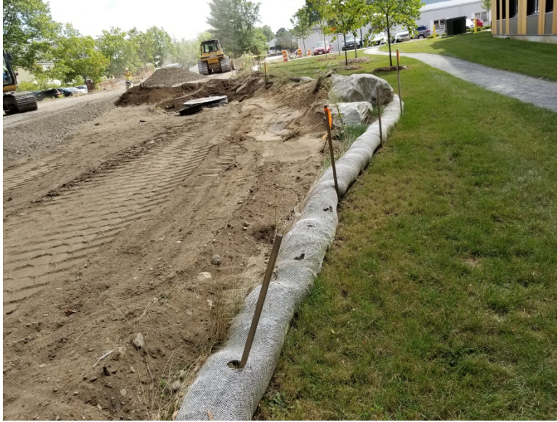
EDGE OF WORK AREA WITH EROSION CONTROL
