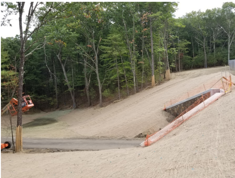
JUTE NETTING AT POWDER MILL RD
