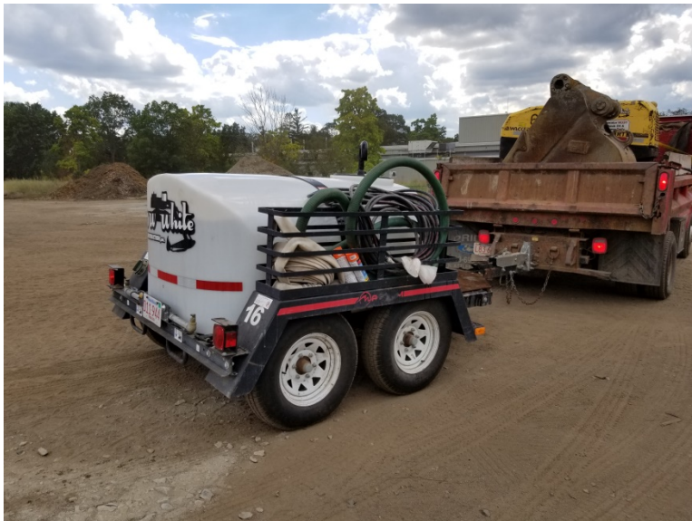
PORTABLE WATER SPRAY FOR DUST CONTROL
