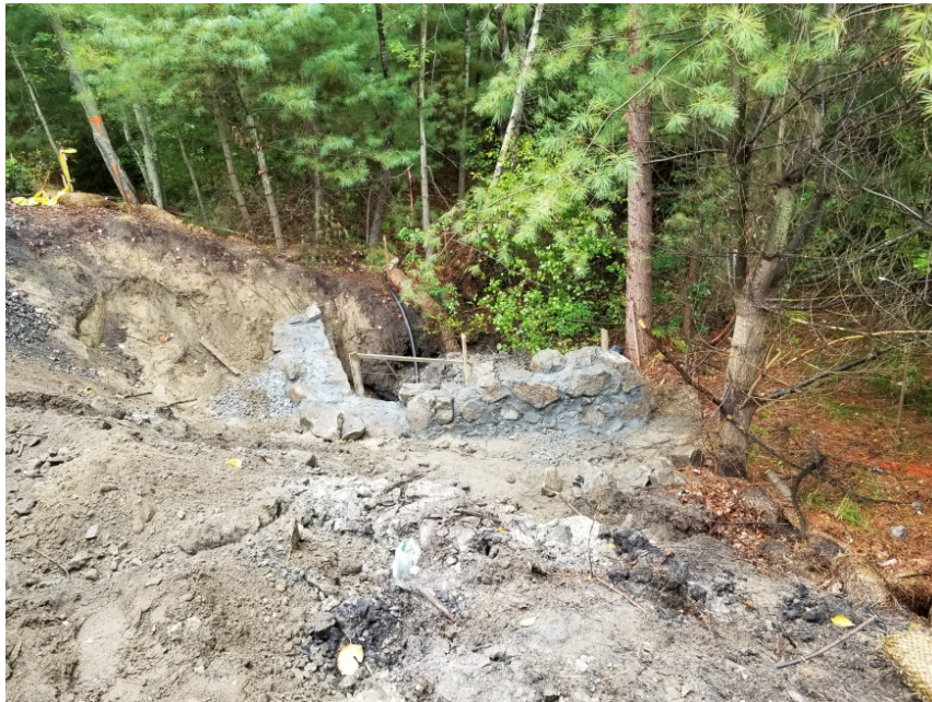
STONE WORK AT CULVERT LOCATED AT STATION 81+10
