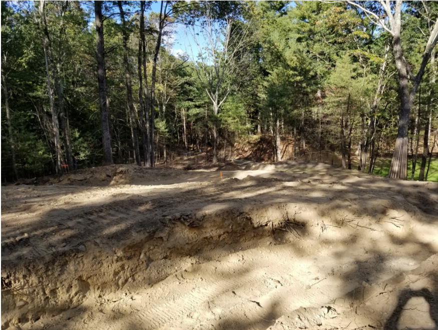
CONSTRUCTION OF PATHWAY BETWEEN TRAIL AND POWDER MILL ROAD
