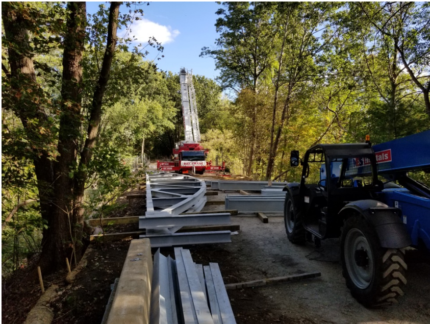
PREPERATION OF BRIDGE #C-19-038
