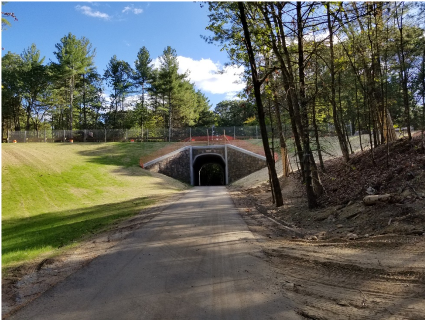
POWDER MILL ROAD CULVERT AND STABILIZATION STATUS
