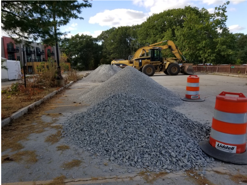
STORAGE OF MATERIAL AND EQUIPMENT
