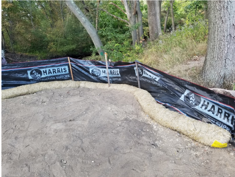
SEDIMENT WASHOUT CORRECTED
