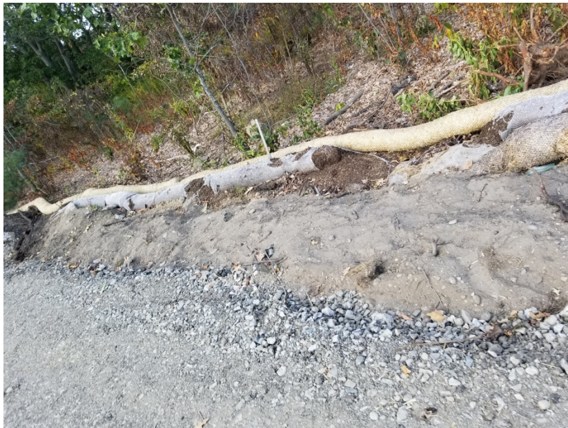
EROSION CONTROL CORRECTED
