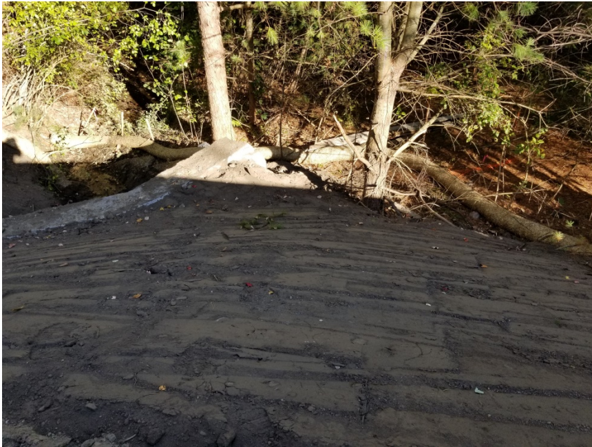
BACKFILL FOR CULVERT LOCATED AT STATION 81+10
