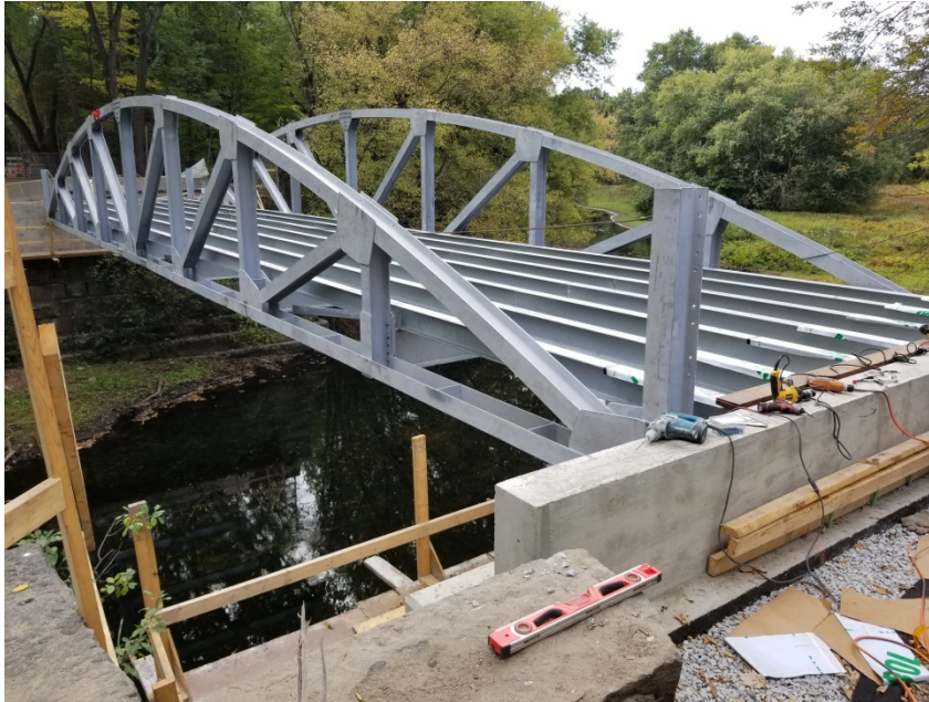
BRIDGE #C-19-038 PLACED UPON THE CONCRETE ABUTMENTS.
