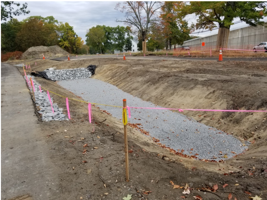
EROSION CONTROL TO BE INSTALLED SURROUNDING DRAINAGE BASIN.
