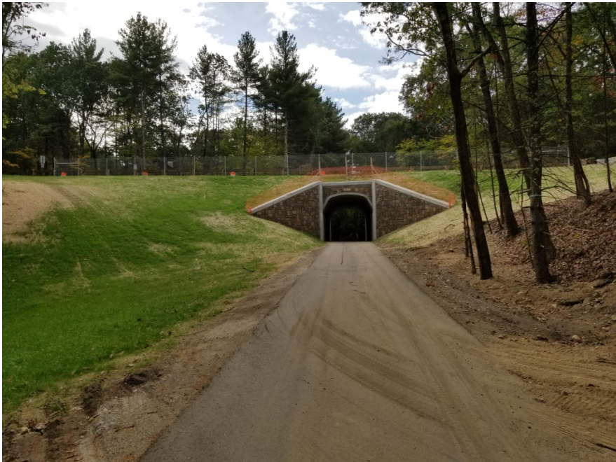
POWDER MILL ROAD CULVERT AND STABILIZATION STATUS
