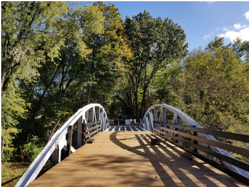
BRIDGE #C-19-038 CURRENT CONDITION.
