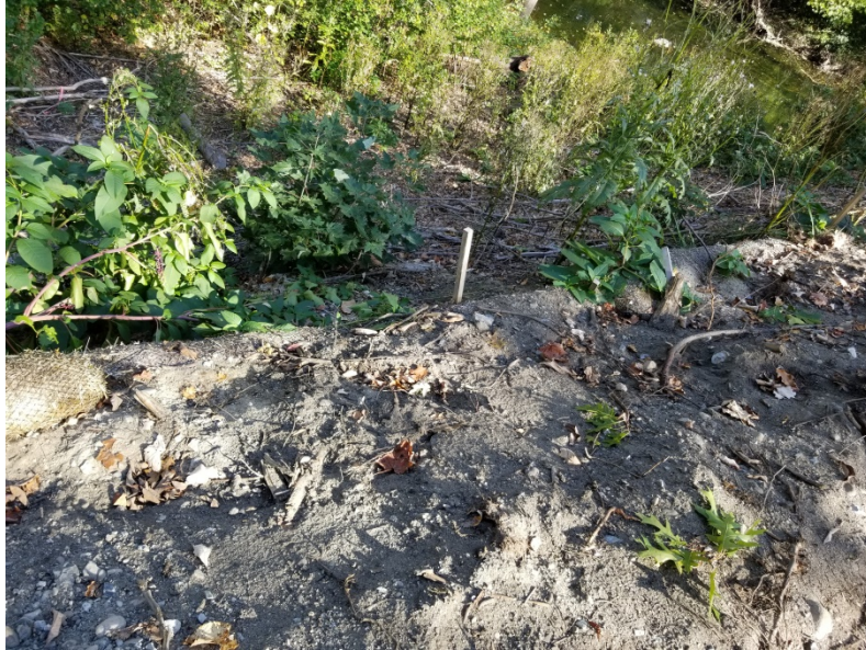
EROSION CONTROL WHICH SHALL BE REPLACED NORTH OF BRIDGE #C-19-038.
