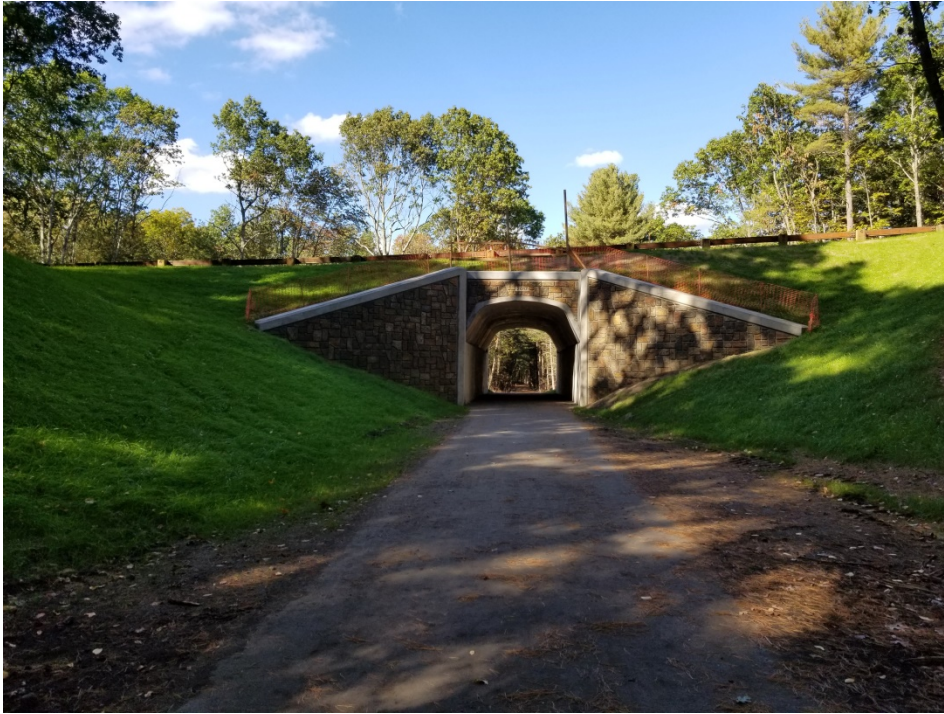
POWDER MILL ROAD CULVERT AND STABILIZATION STATUS
