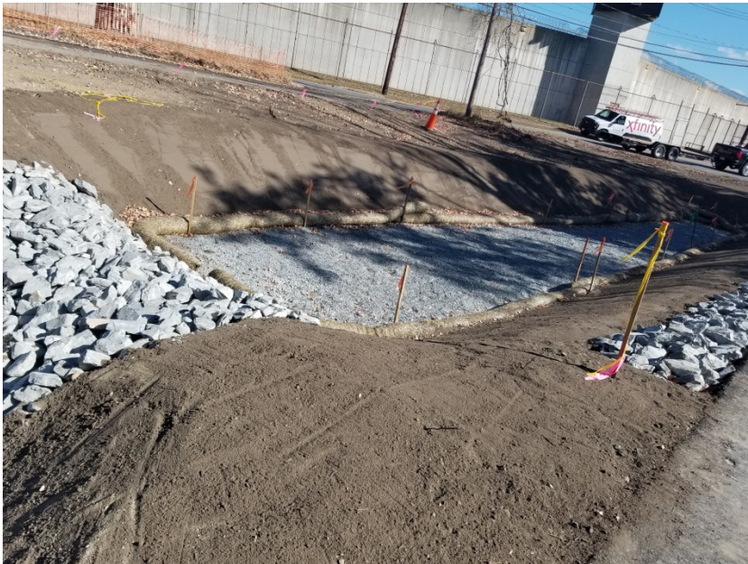
EROSION CONTROL INSTALLED SURROUNDING DRAINAGE BASIN.
