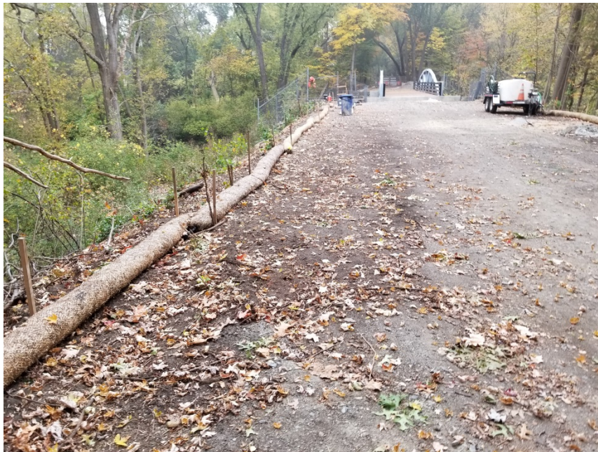
EROSION CONTROL REPLACED NORTH OF BRIDGE #C-19-038.
