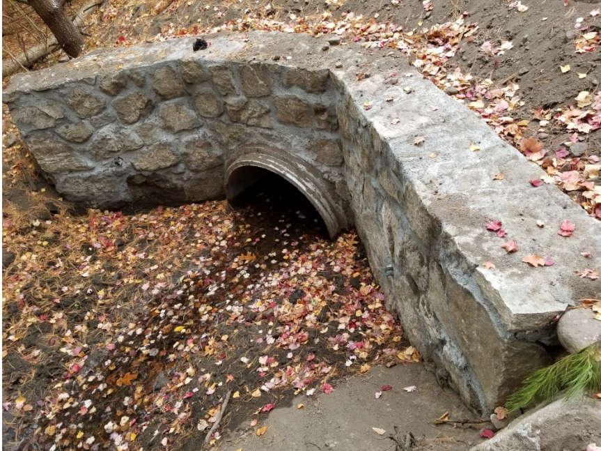
CULVERT AT STATION 81+10 STATUS
