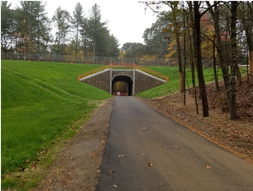
POWDER MILL ROAD CULVERT AND STABILIZATION STATUS
