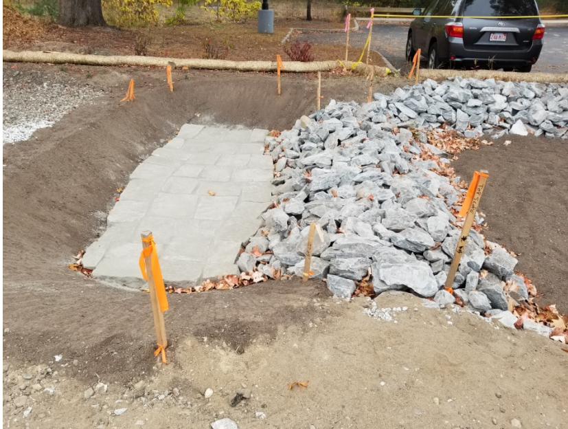
STONE BASE ON FOREBAY INSTALLED.
