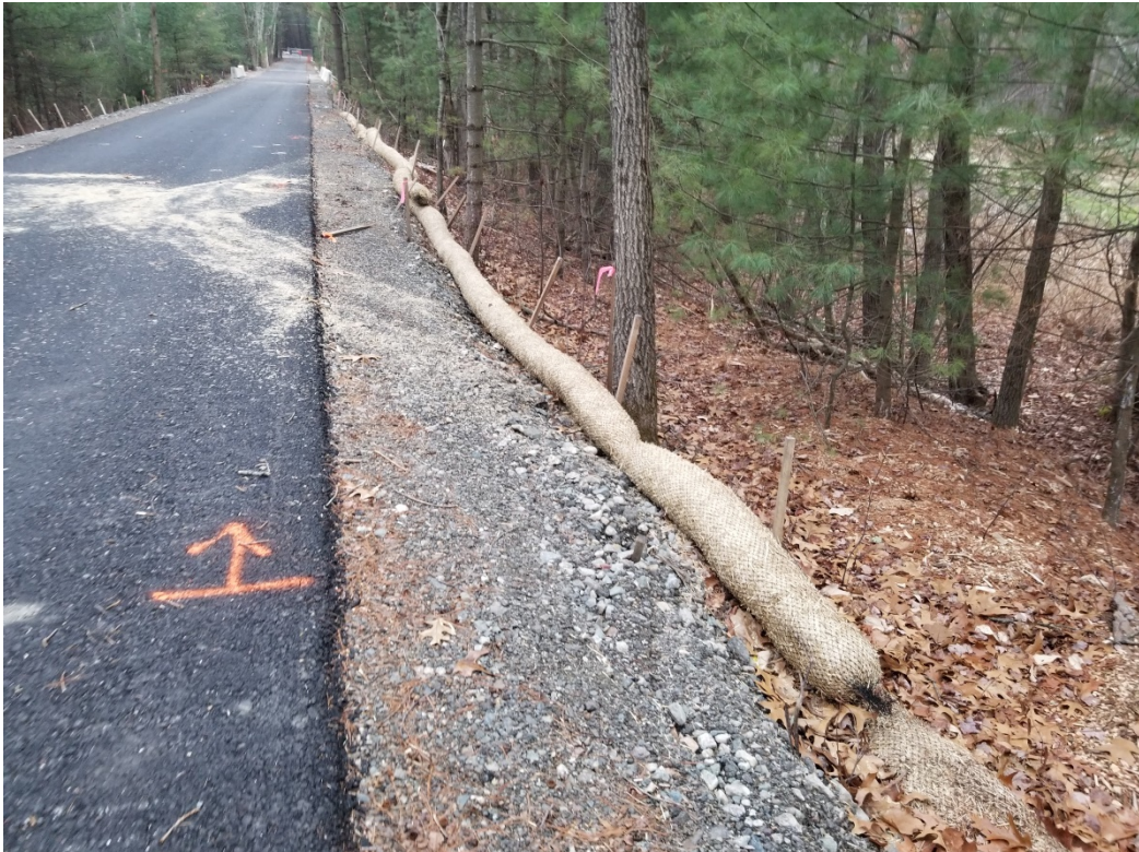
EROSION CONTROL WHICH WAS REPLACED AND REPAIRED.
