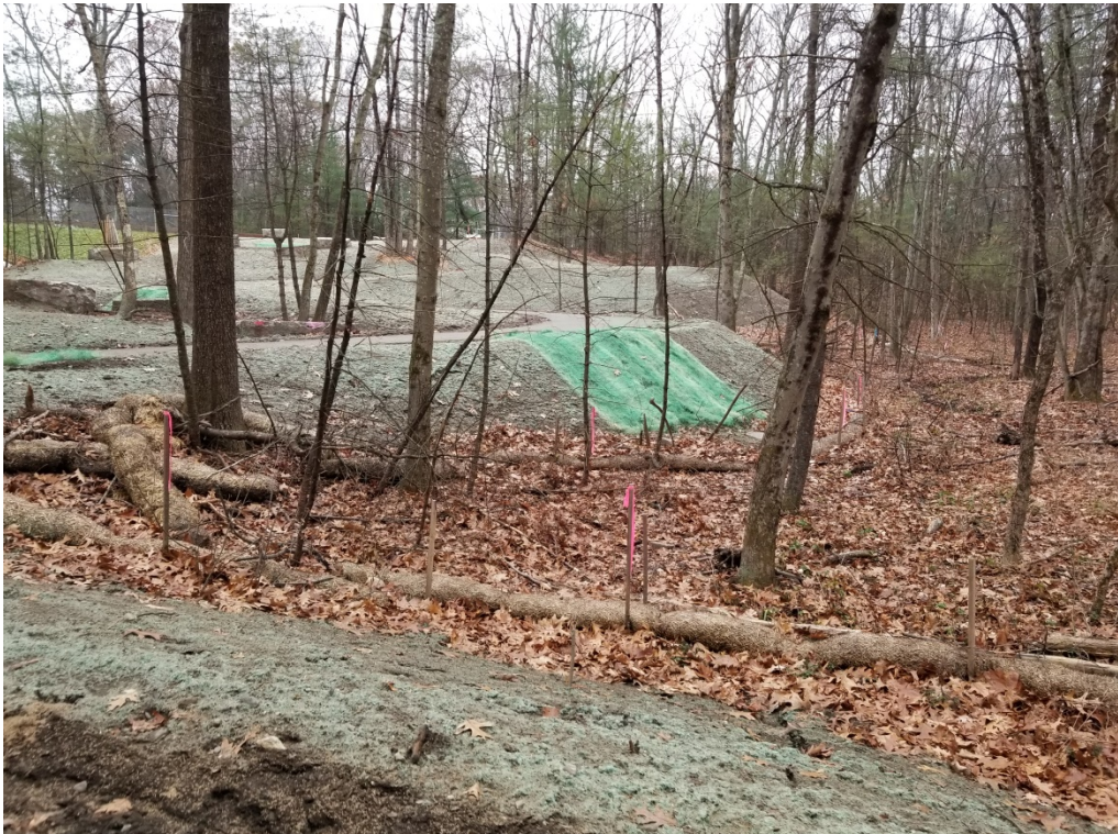
SEDIMENT WASHOUT REPAIRED LOCATED AT POWDER MILL ROAD HANDICAP RAMP.
