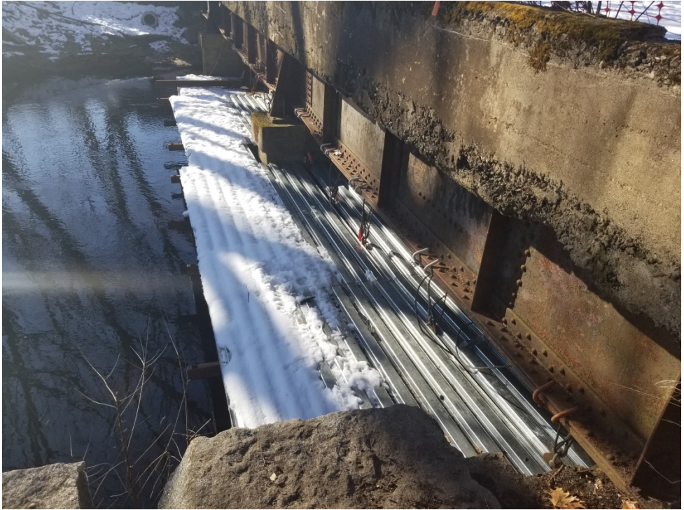
STATUS OF THE SAFTEY PLATFORM LOCATED AT THE REHABILITATION BRIDGE.
