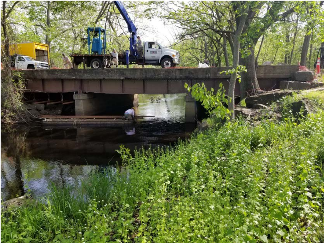
REHABILITATION BRIDGE NEAR BROOKSIDE SQUARE AFTER PAINTING HAS FINISHED.
