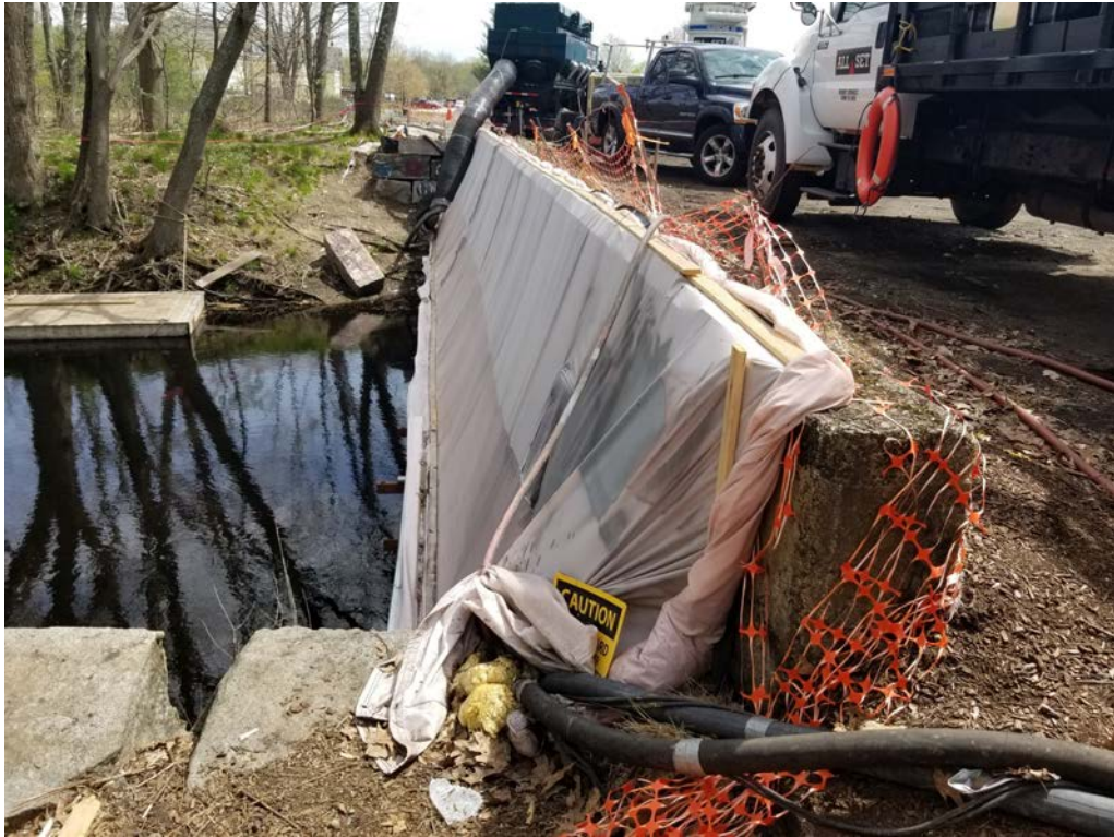
REHABILITATION BRIDGE NEAR BROOKSIDE SQUARE WHILE SAND BLASTING HAS COMMENCED.
