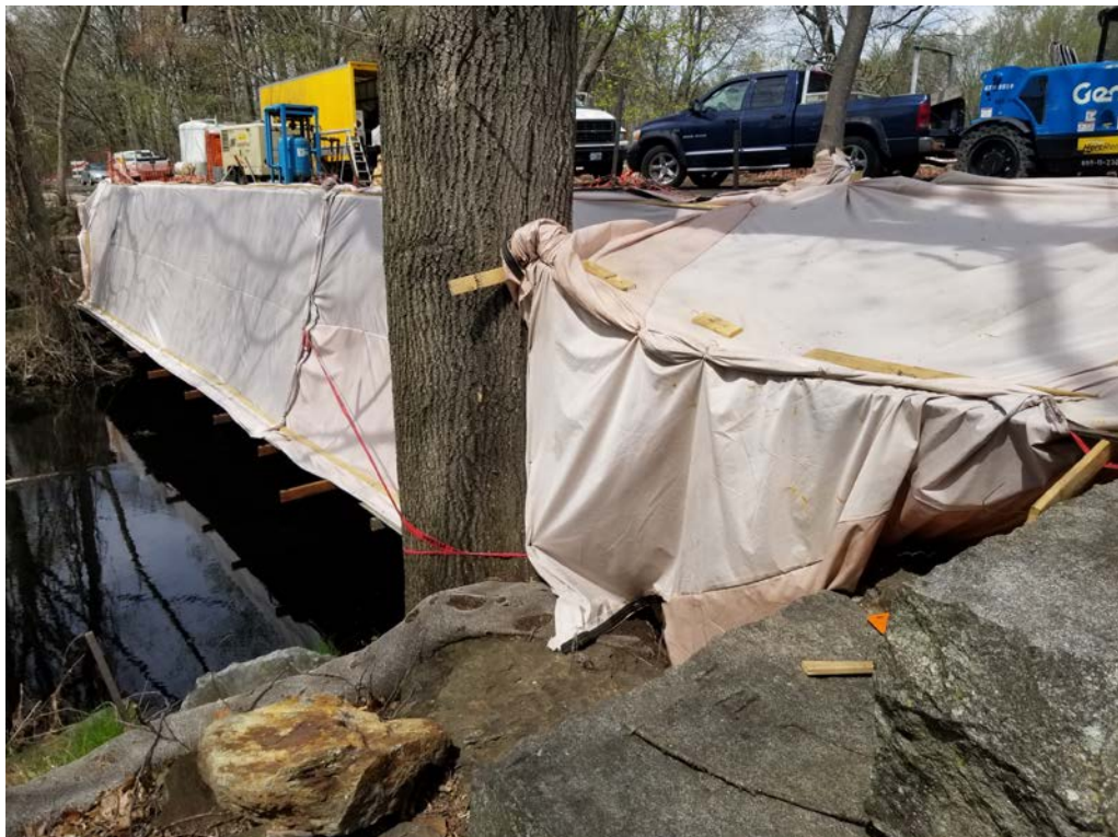
REHABILITATION BRIDGE NEAR BROOKSIDE SQUARE.
