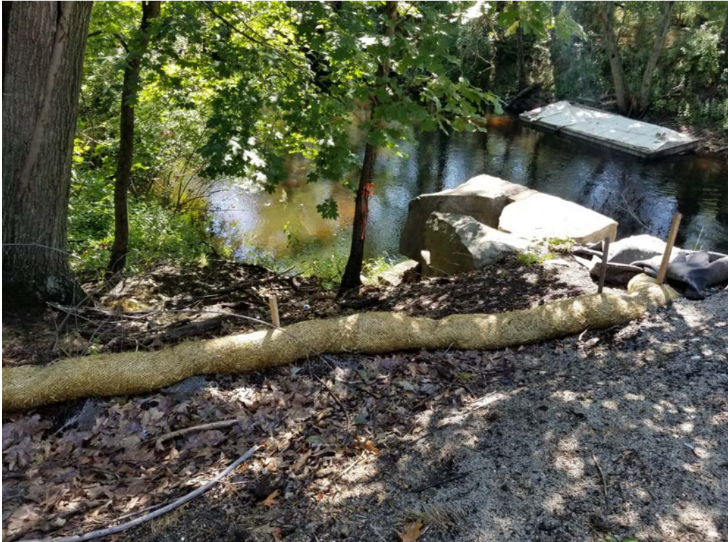
REHABILITATION BRIDGE (C-19-036) NEAR BROOKSIDE EROSION CONTROL ADDED.
