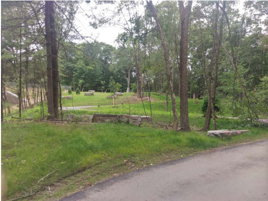
POWDER MILL ROAD PATHWAY AFTER REPAIRS AND RAINFALL.
