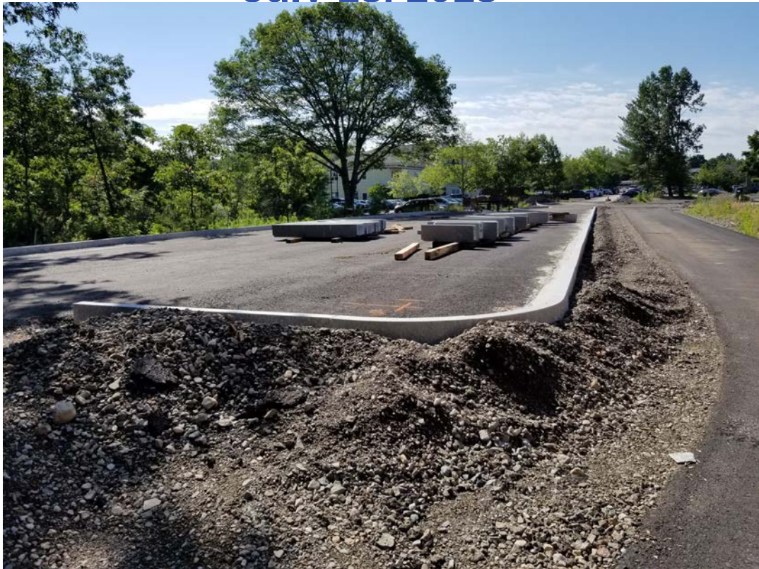
CURBING ADDED TO PARKING LOT NEAR BROOKSIDE SQUARE.
