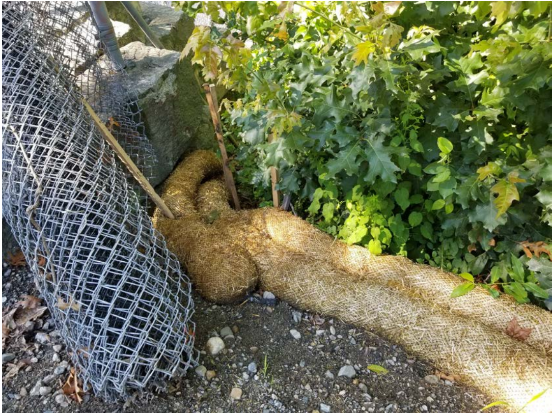
EROSION CONTROL ADDED ALONG BRIDGE #19-038.
