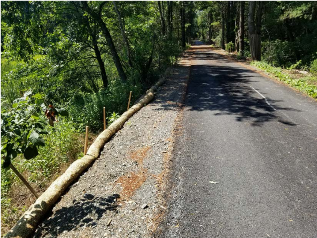
EROSION CONTROL INSTALLED BETWEEN STATION 65 AND 50.
