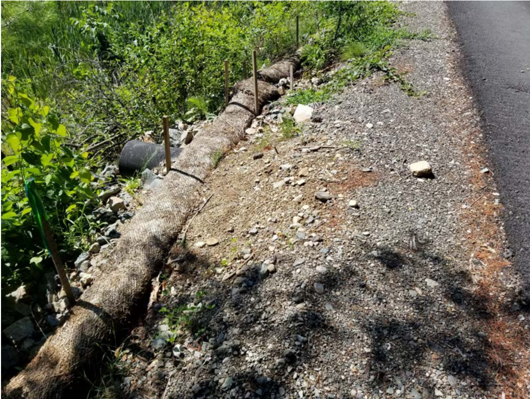
SEDIMENT REMOVED BETWEEN STATION 65 AND 50.
