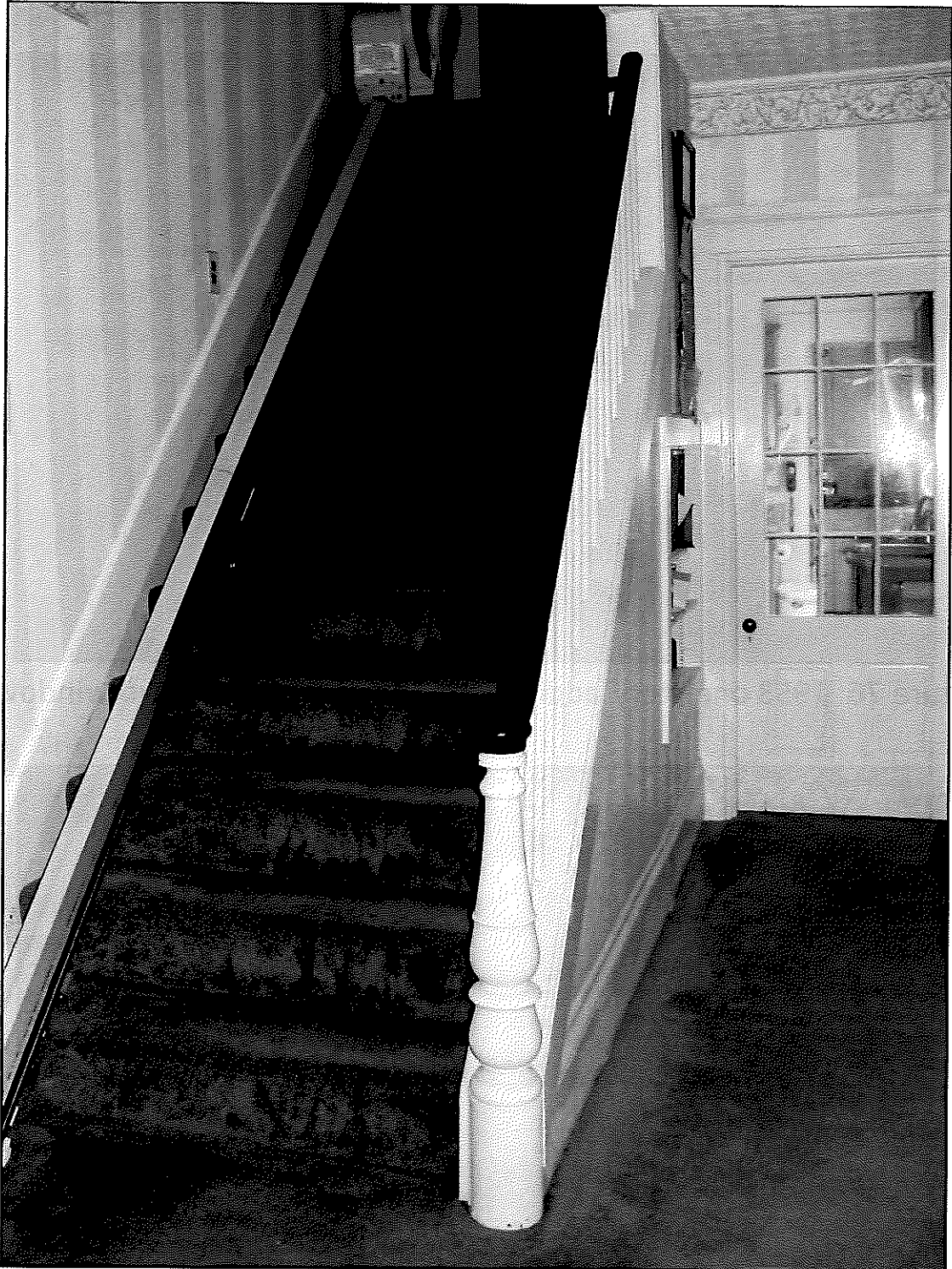
Figure 78: Rebuilt back stair to second floor, widened in 1977, newel post and railing salvaged from original stair (Original door w/ glass to kitchen seen at right, at end of back hallway)
