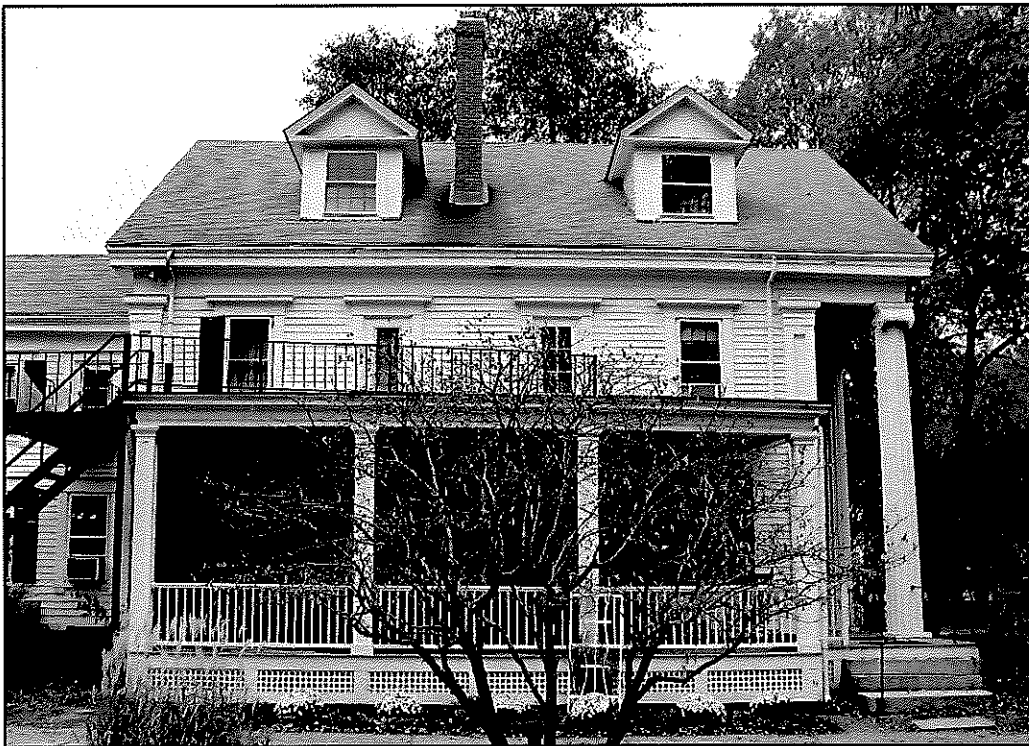
Figure 72: Porch at east side of main house
