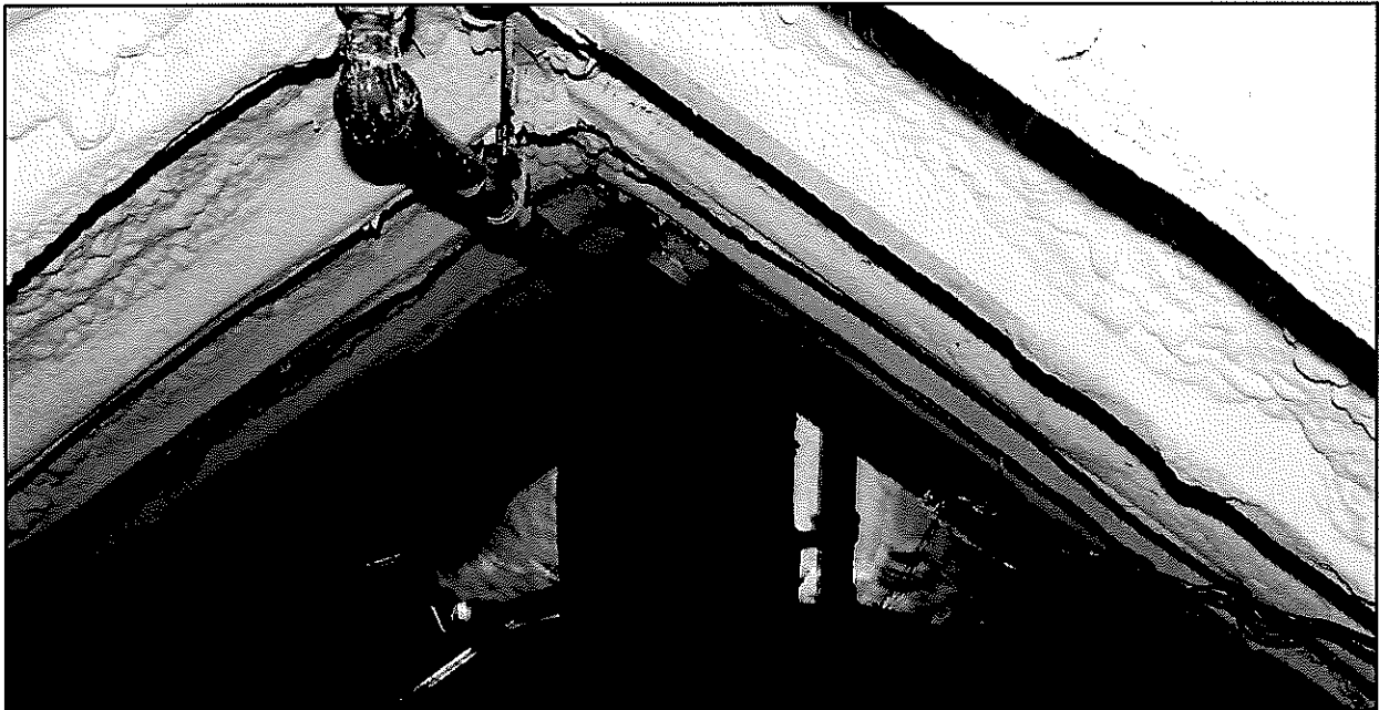
Figure 19: Ell roof rafters, sprayed with insulated foam
