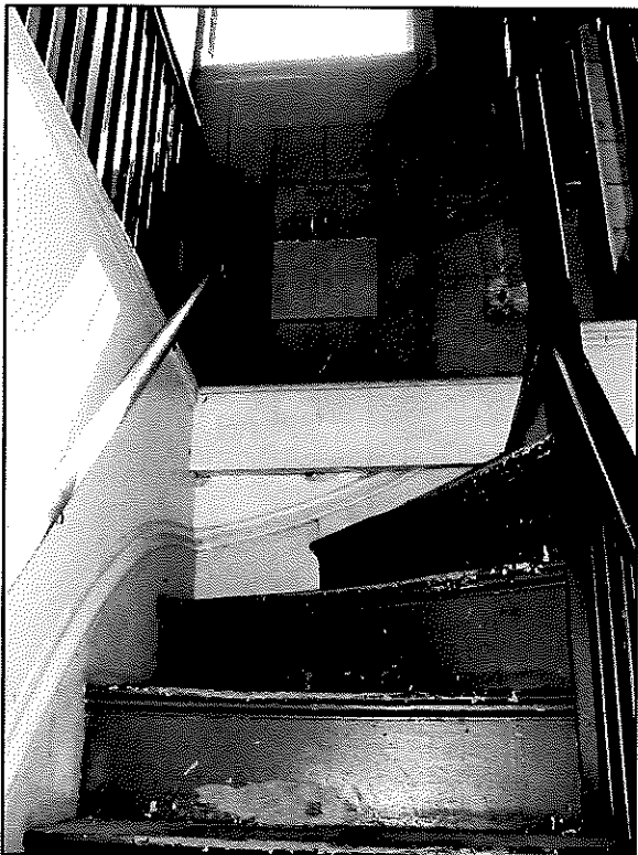
Figure 51: Stair up to attic and its lower newel post against door jamb
