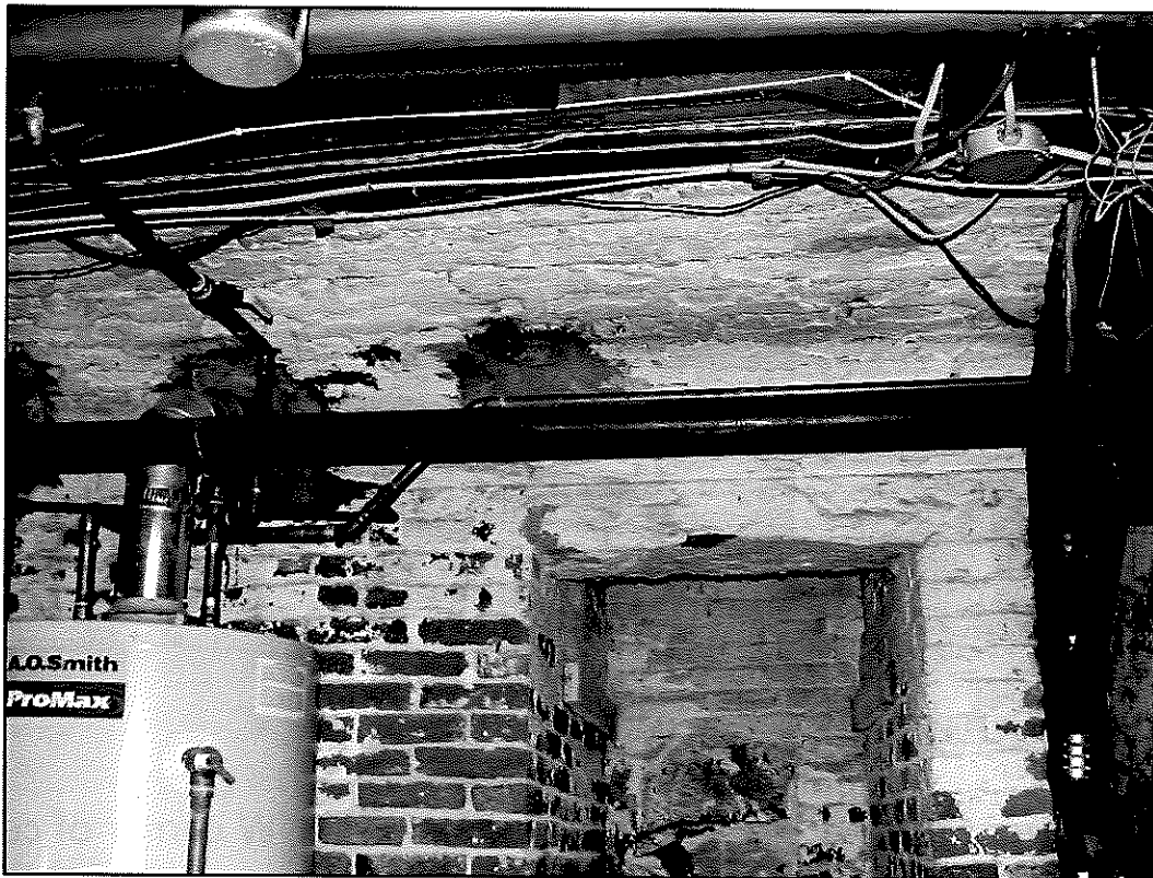
Fig 58: Foundation for ell fireplace and chimney
