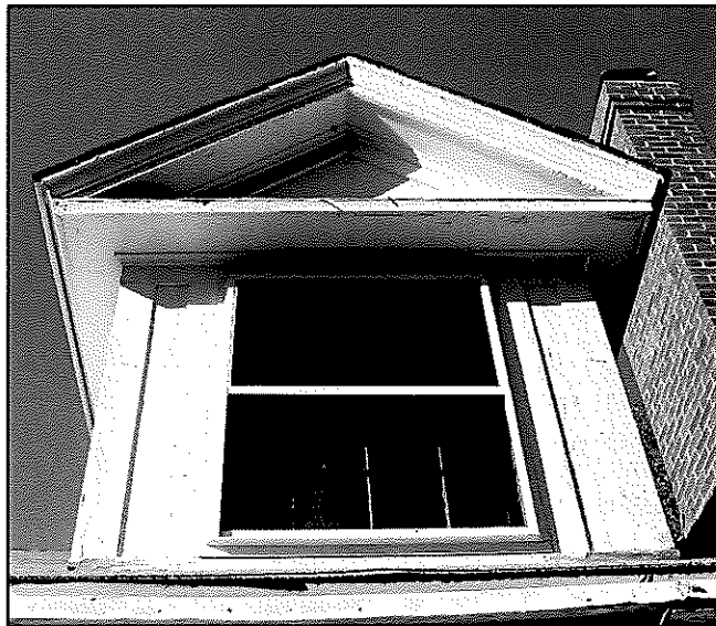
Figure 65: Southeast roof dormer
