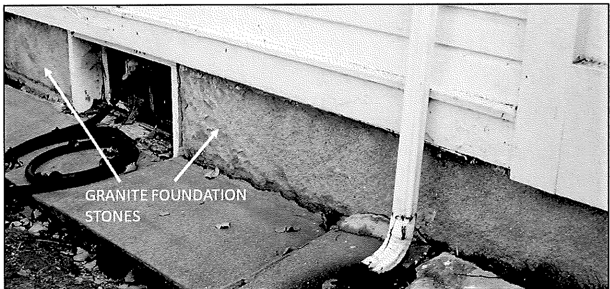
Figure 11: Granite blocks at top of foundation, west exterior wall
