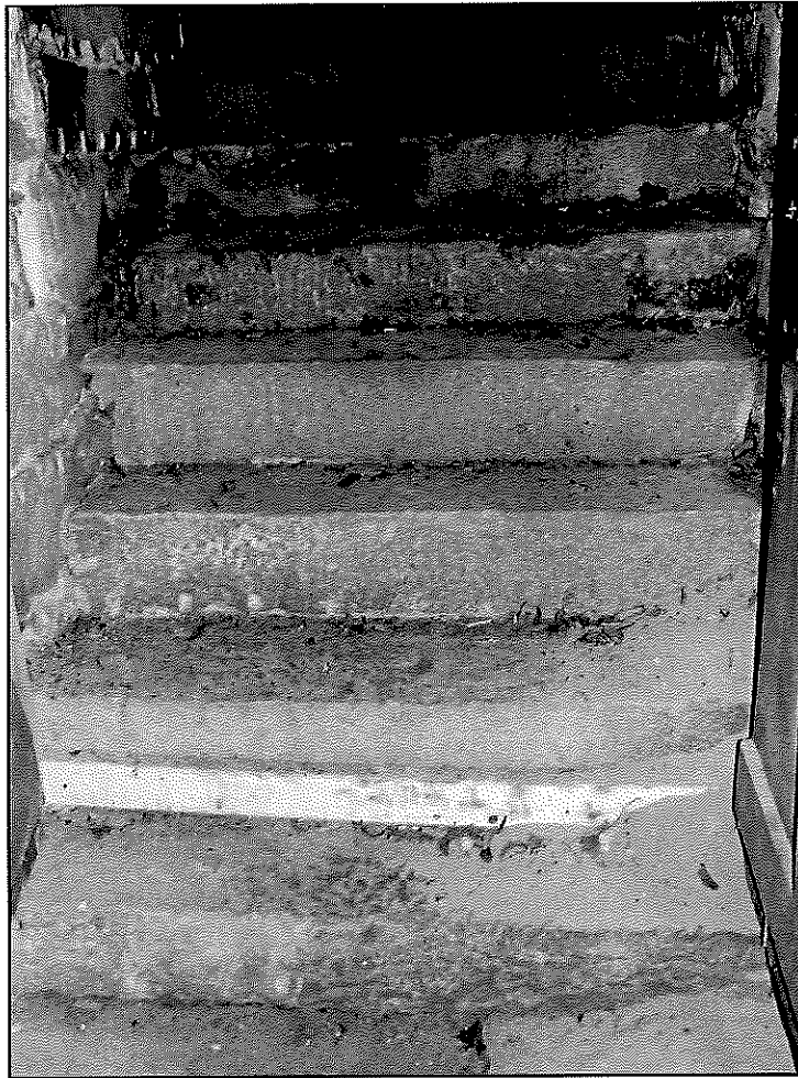
Figure 59: Granite bulkhead stairs (see also fig. 35)
