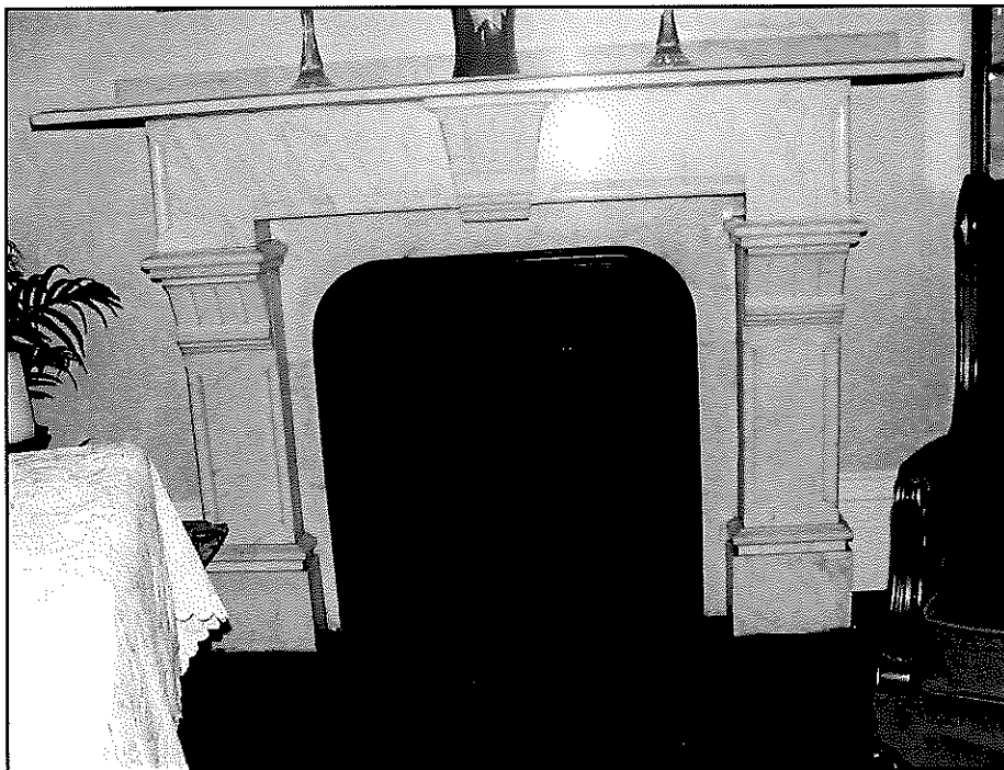
Figure 45: Marble fireplace mantel, 1 st floor, northwest room
