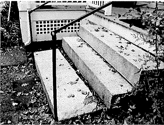
GRANITE STEPS TO PORTICO, OUT OF ALIGNMENT
