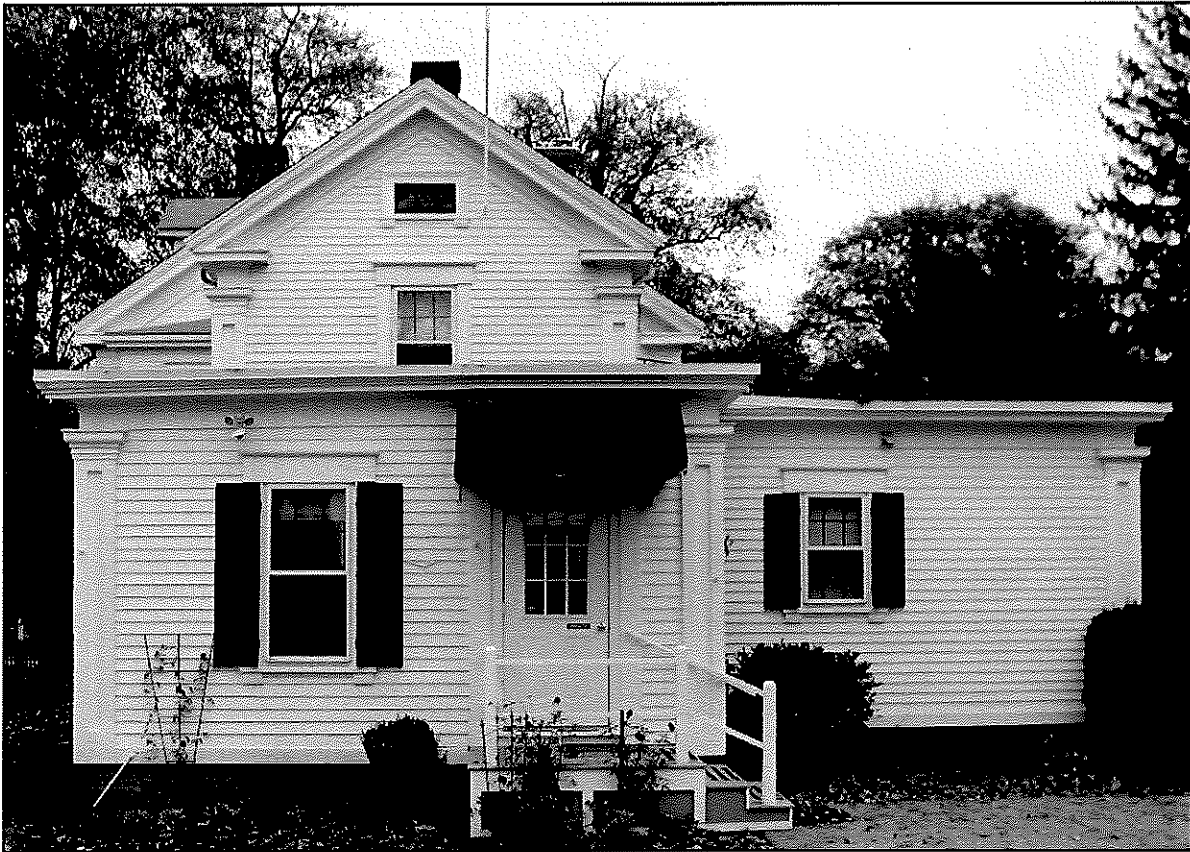
Figure 32: South wall of ell (with later one-story additions), showing original 2 nd floor window, and attic window in gable.
