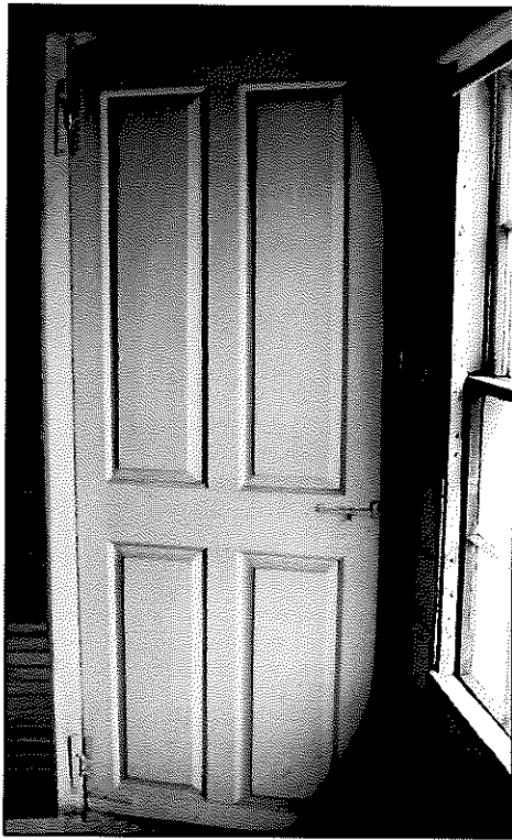
Figure 20: Re-used 18 th -century door w/ H-L hinges at head of attic stair (left) & thumb-latch on opposite side of door (right)
