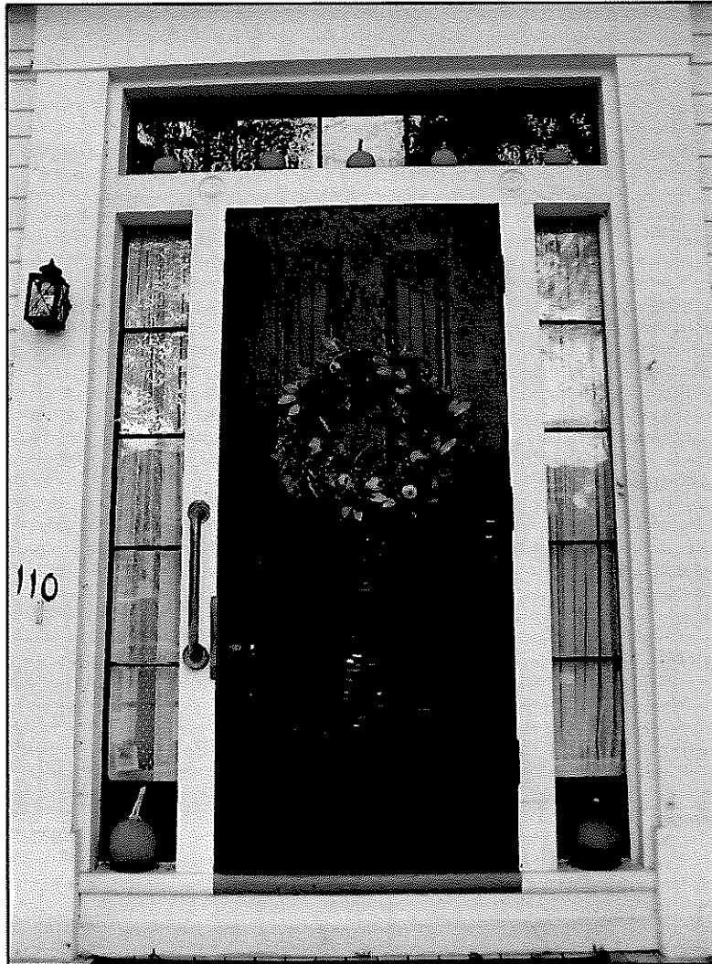
Figure 25: Front door with sidelights and transom sash.
