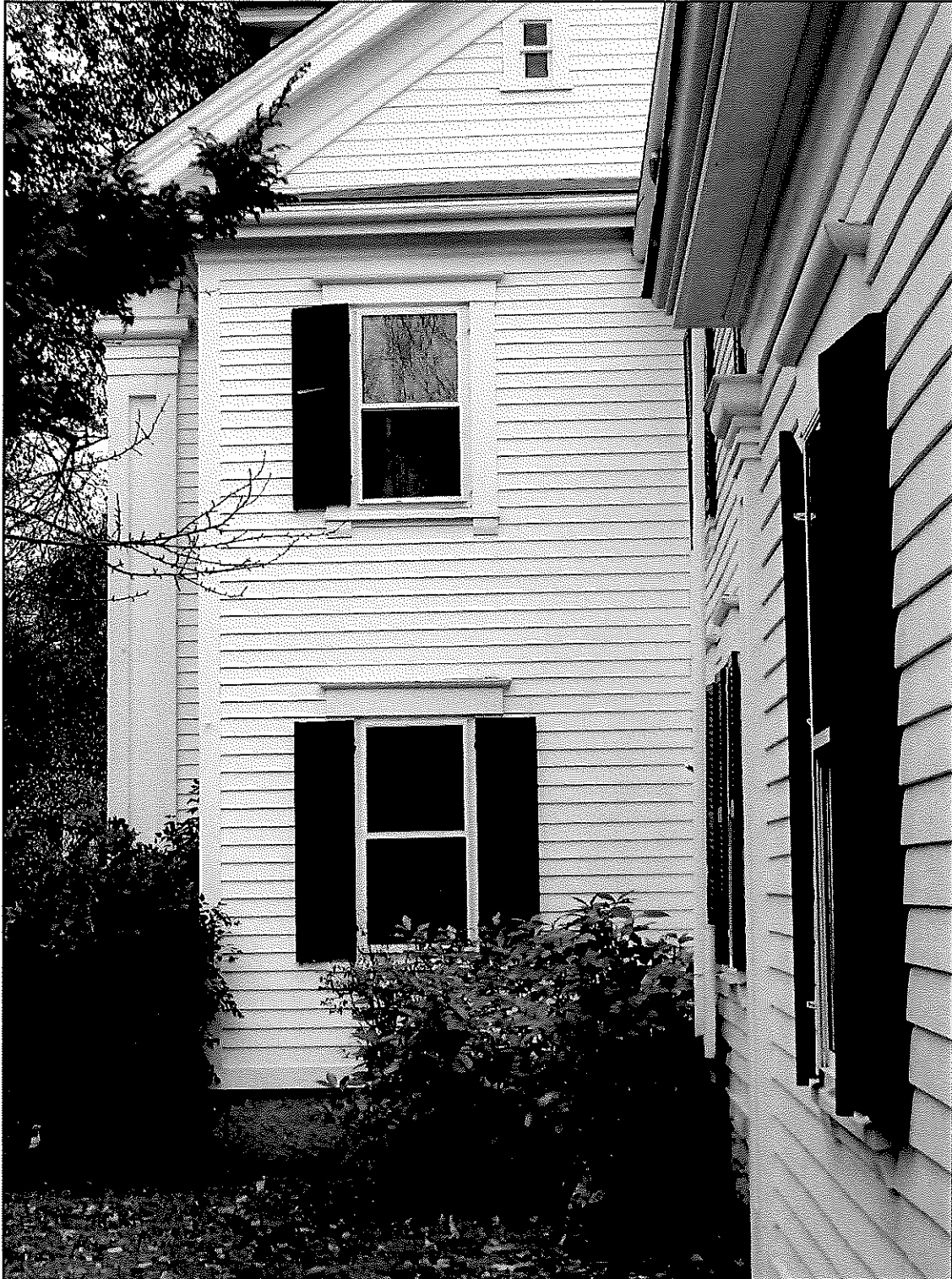
Figure 79: Two-story addition built in two phases against the south wall of main house and its intersection with the west wall of the ell (at right)
