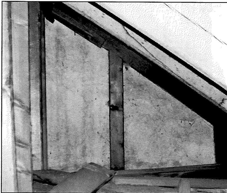
Figure 55: Back plastering between studs in attic, north gable wall
