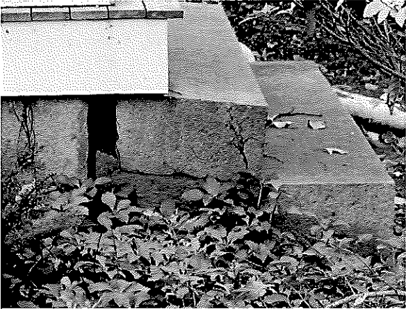
GRANITE STEPS TO PORTICO, OUT OF ALIGNMENT
