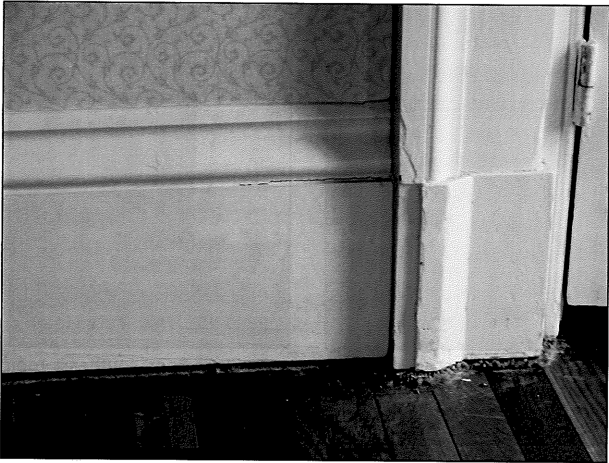
Figure 42: Plinth block at bottom of door architrave and baseboard
