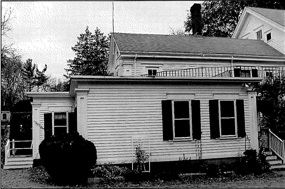
Figure 76: 1953 one-story addition (in foreground with two windows)
