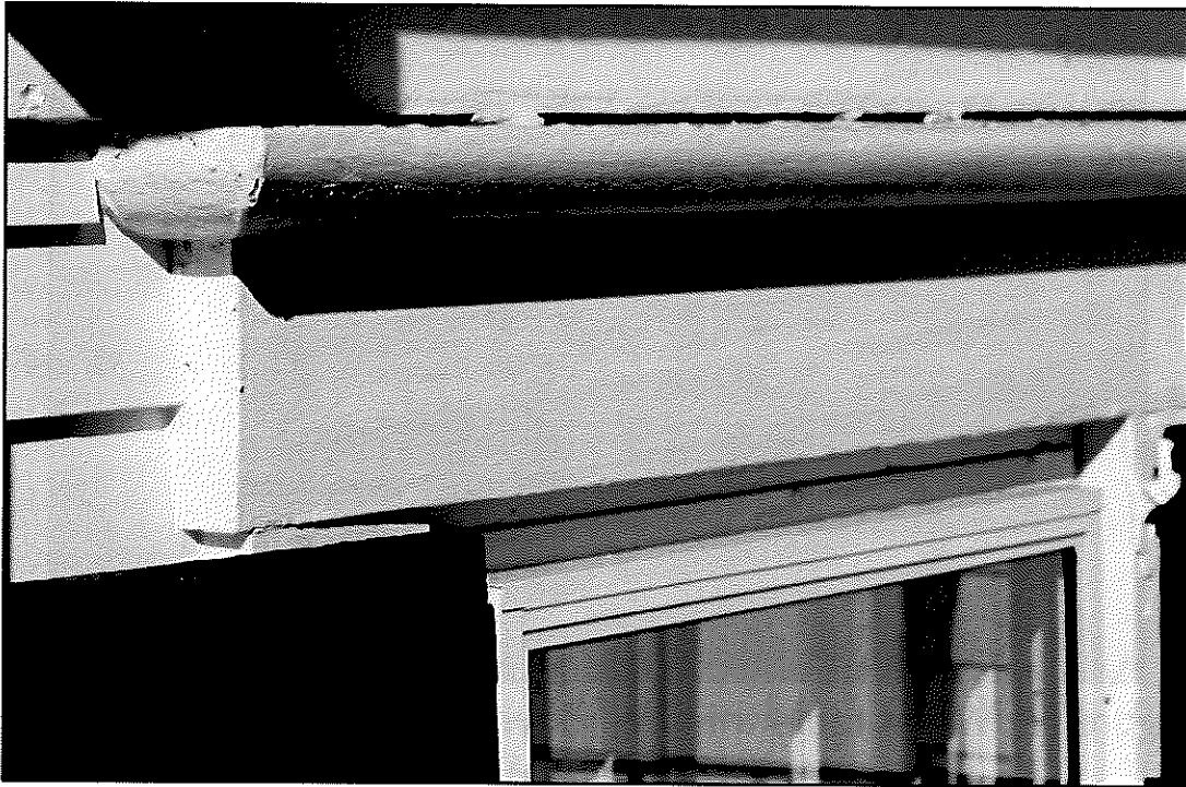
Figure 30: Window cap detail typical for ell windows
