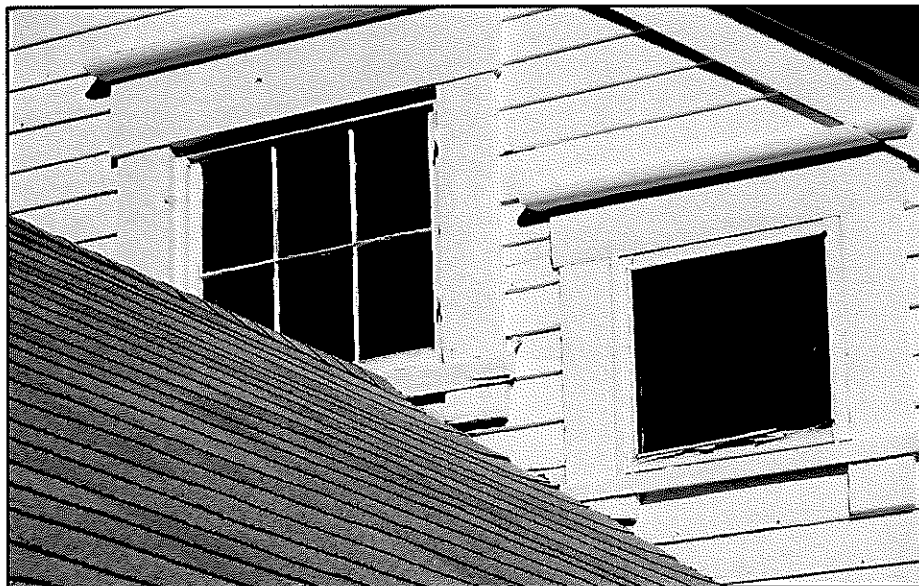
Figure 33: Intersection of ell roof peak at sill of attic window of main house (window at right is a later addition)
