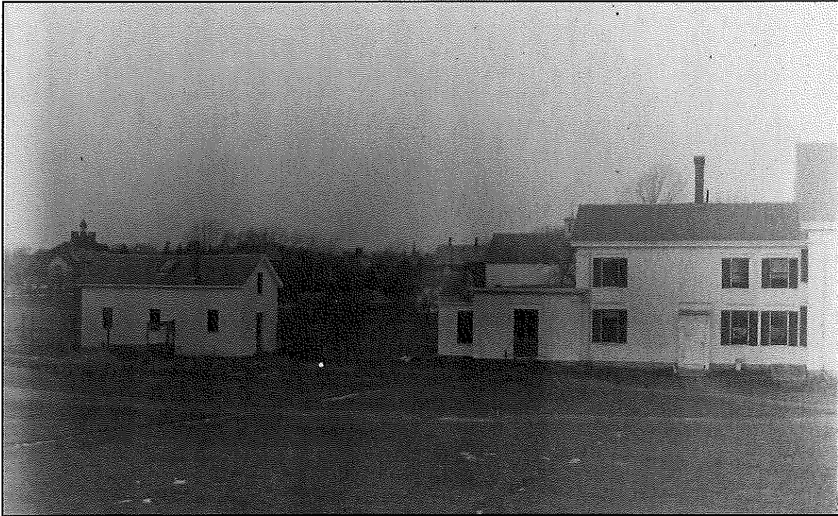
Figure 8: Everett family photo of 110 Walden Street, looking west, showing the rear ell and additions, ca. 1880 Courtesy Concord Free Public Library
