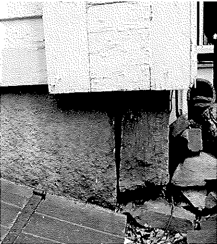
OPEN JOINTS IN FOUNDATION STONES
