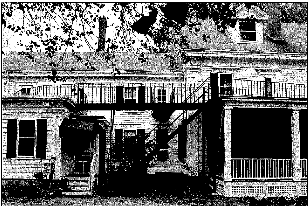
Figure 77: Small porch (behind green awning) at side entrance to ell and metal fire escape bridge and stair
