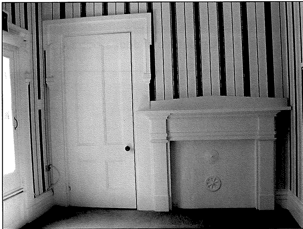
Figure 41: Window, door and mantel trim, 2 nd floor, northeast room
