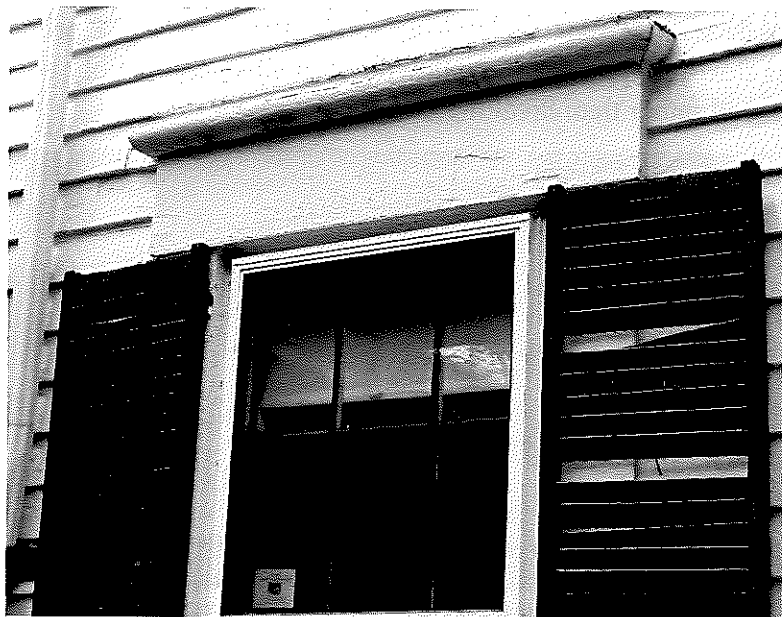
LOUVERS FALLING OUT OF BLIND FRAMES
