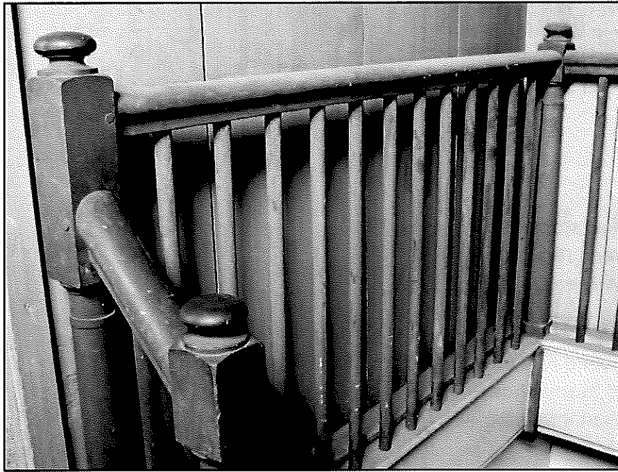
Figure 52: Upper newel posts and balustrade within vertical board enclosure at attic level
