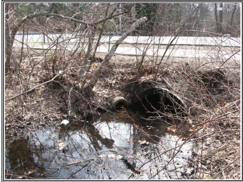
Photograph No. 7: Watershed Reconnaissance W-15 culvert at Lawson Brook Road
