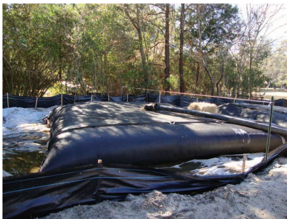
Geotubes used to dewater hydraulically dredged material
