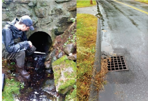
Measuring flow from outfall and stormwater discharging to a catch basin on Wright Road during wet weather sampling.
