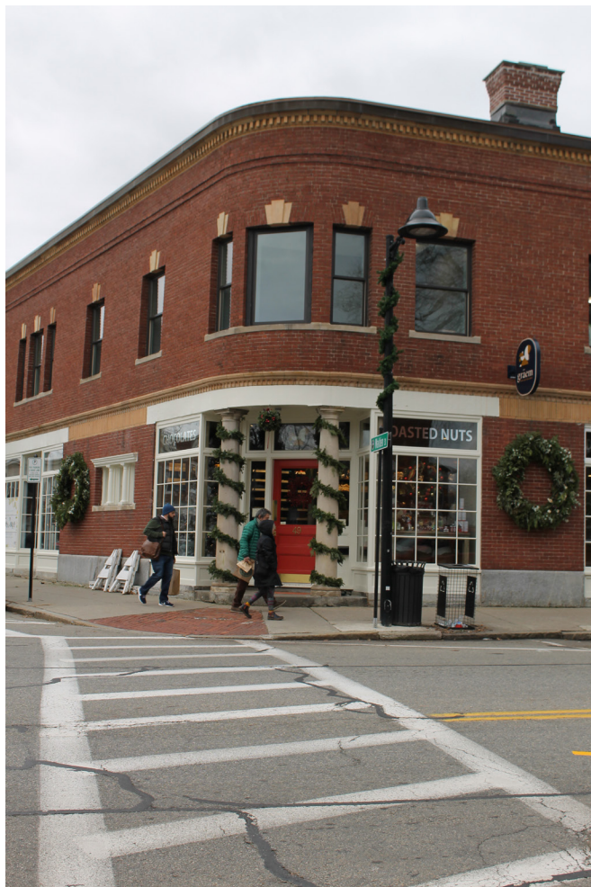
The Friend Building – renovated and opened in 2018 with Graem Nuts and Chocolates and Caffè Nero
