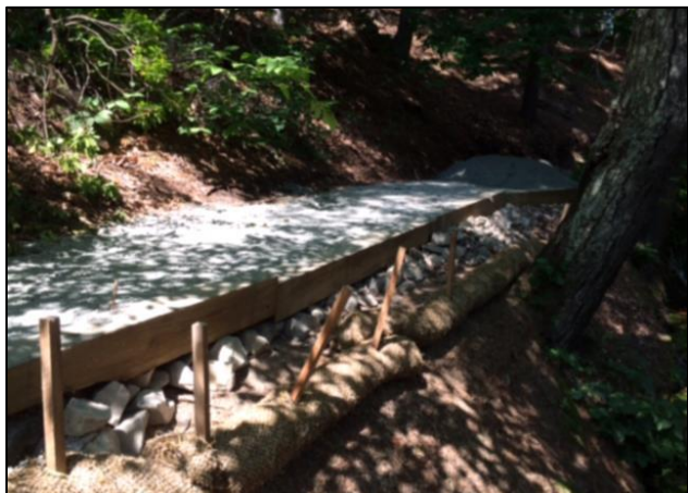
Installation of regraded gravel trail with timber curbing (left) and and bioretention area (right).
