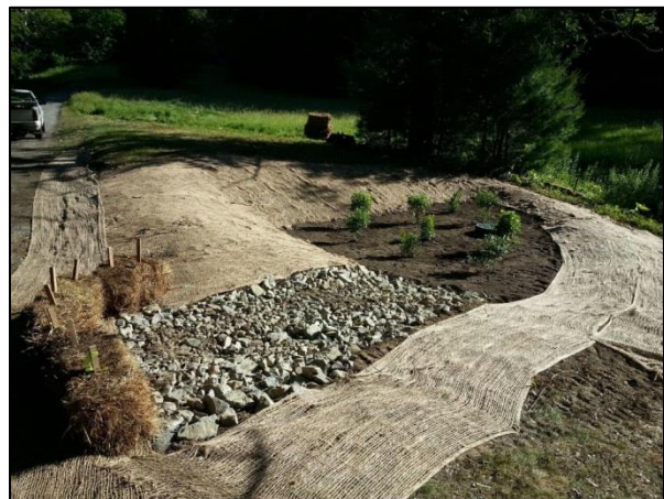
Installation of regraded gravel trail with timber curbing (left) and and bioretention area (right).
