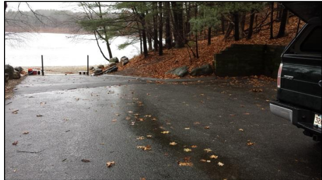
Stormwater flowing down the public access boat launch is partially captured by infiltrating catch basins. Water not captured by these catch basins is able to flow straight down to the pond.
