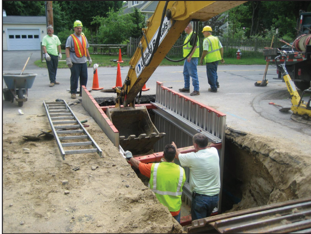
Drainage project on Whittemore Street
