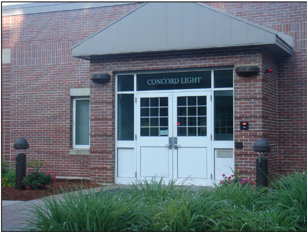
Concord Municipal Light Plant, 1175 Elm Street
