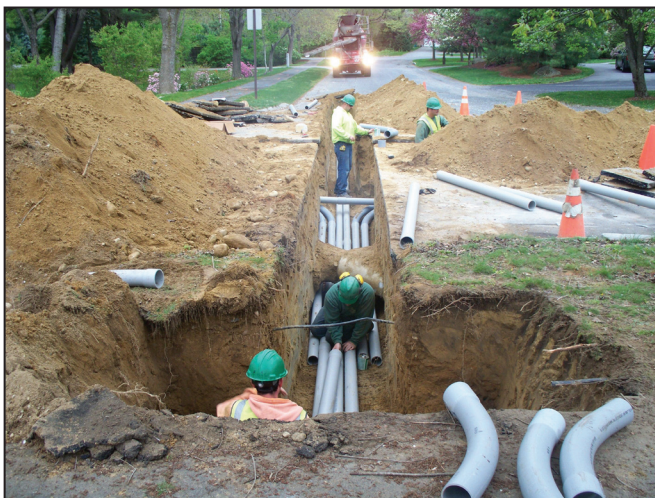
Construction workers install conduits under a drain line for underground electric cables on Mildred Circle.
