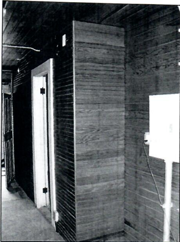
Figure 67: Two types of "bead-board" sheathing used in attic hallway
