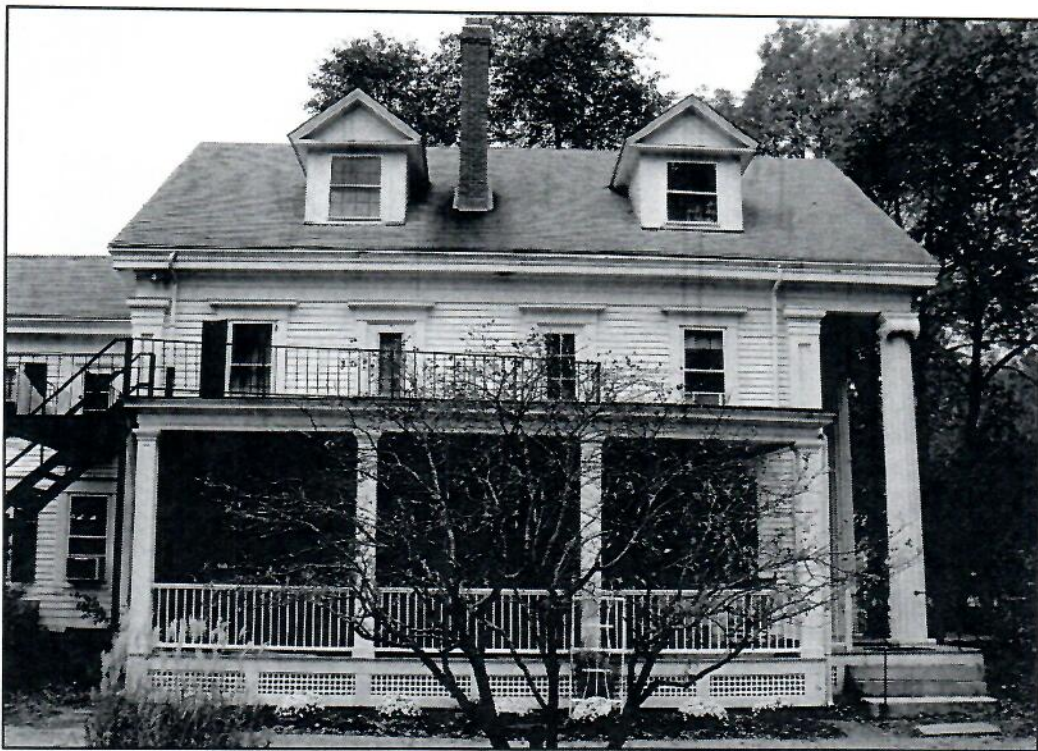
Figure 72: Porch at east side of main house
