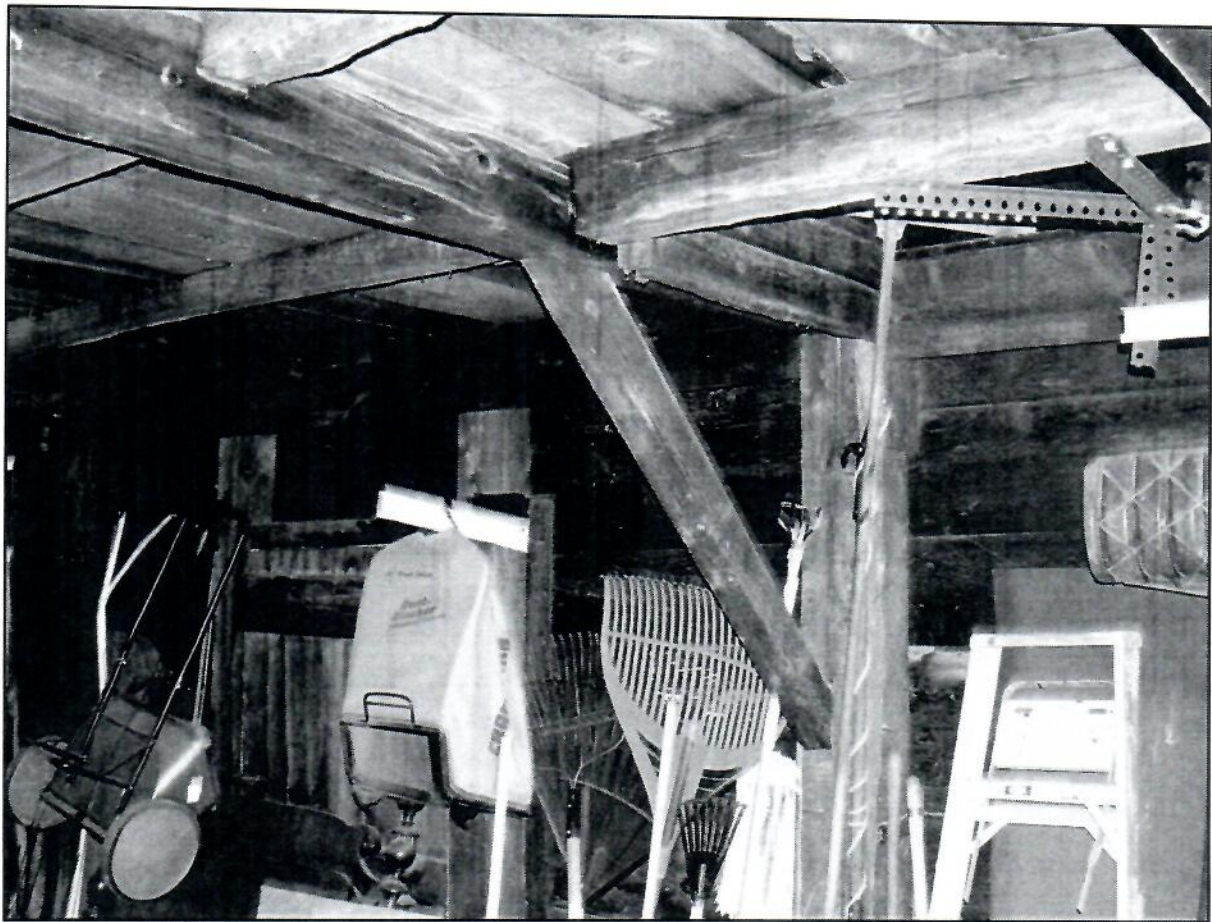
Figure 62: Post and beam framing inside shed
