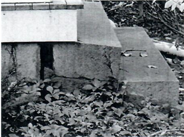
GRANITE STEPS TO PORTICO, OUT OF ALIGNMENT
