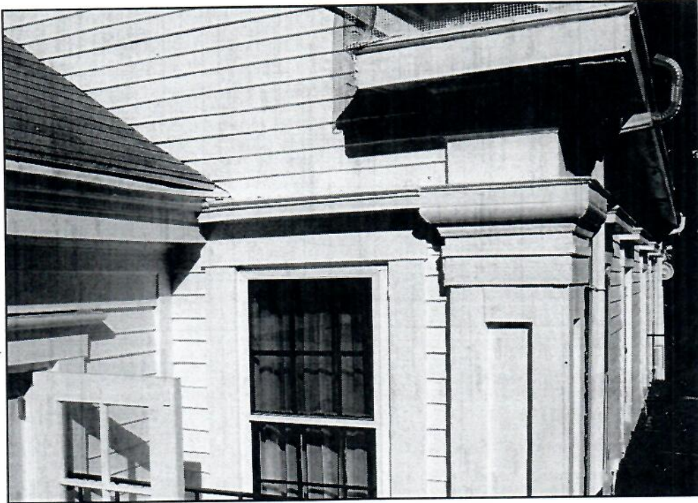
Figure 34: Intersection of ell roof east eaves with 2 nd floor window cap at main house south wall, southeast corner
