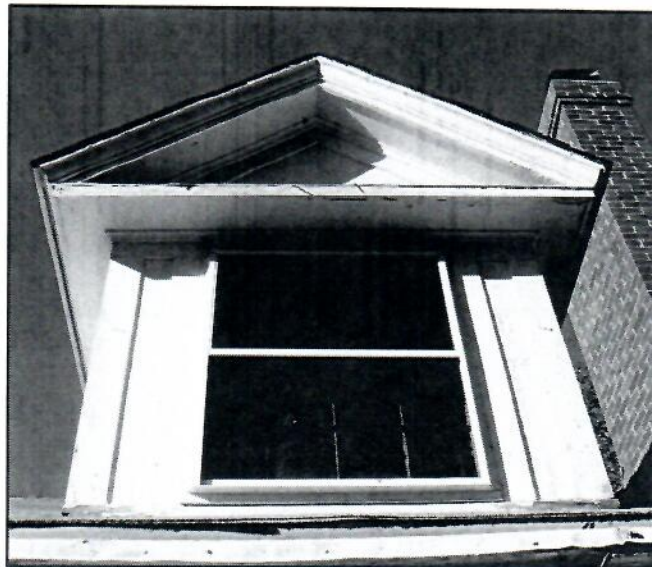
Figure 65: Southeast roof dormer
