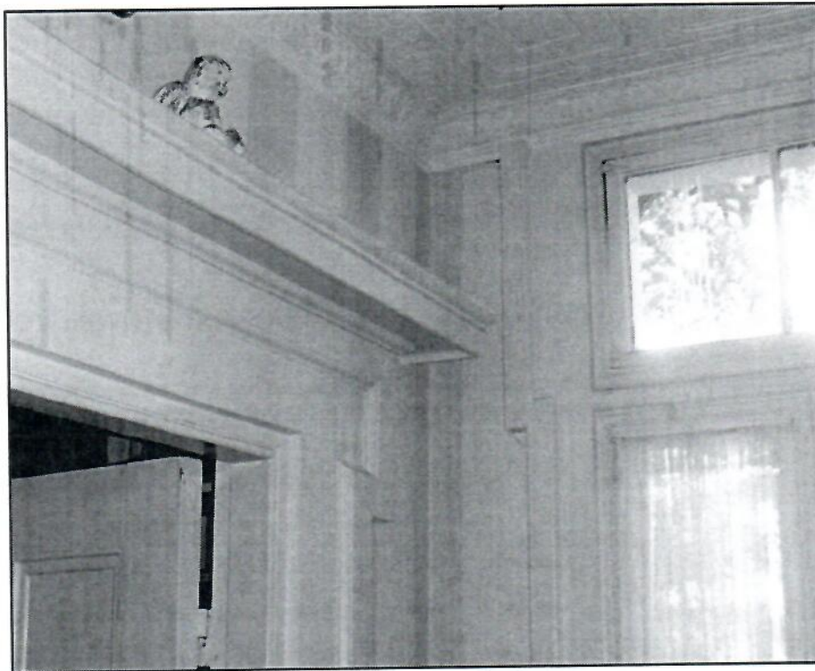
Figure 38: Door architraves and headers, 1 st floor, front hall
