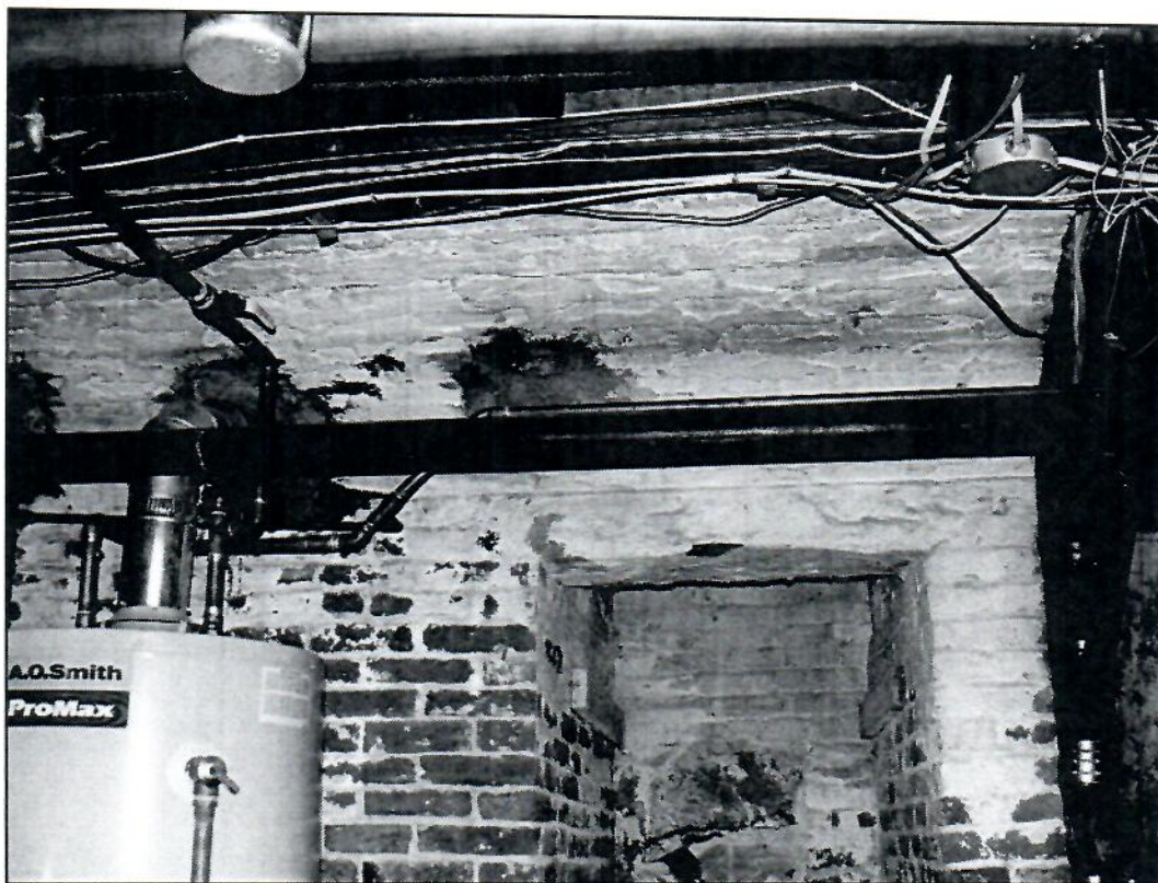
Fig 58: Foundation for ell fireplace and chimney
