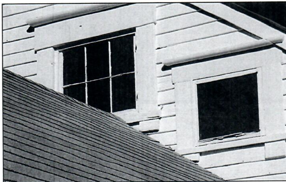
Figure 33: Intersection of ell roof peak at sill of attic window of main house (window at right is a later addition)
