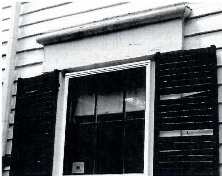
LOUVERS FALLING OUT OF BLIND FRAMES
