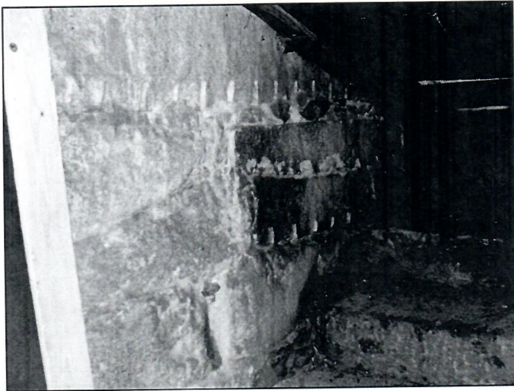
Figure 35: Granite bulkhead wall and stairs to cellar
