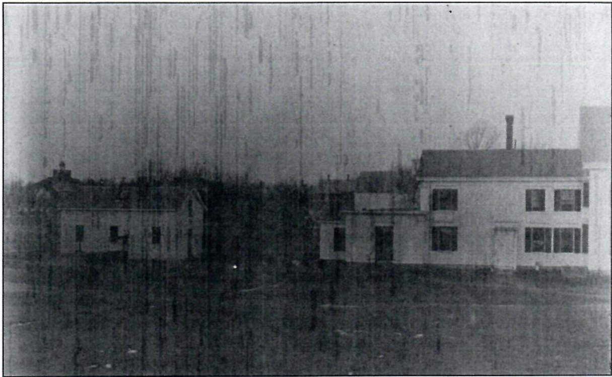
Figure 8: Everett family photo of 110 Walden Street, looking west, showing the rear ell and additions, ca. 1880
