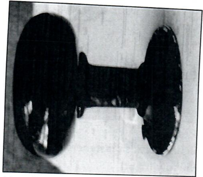
Figure 48: Glass knob with silver backing (left) & mineral knob (right)
