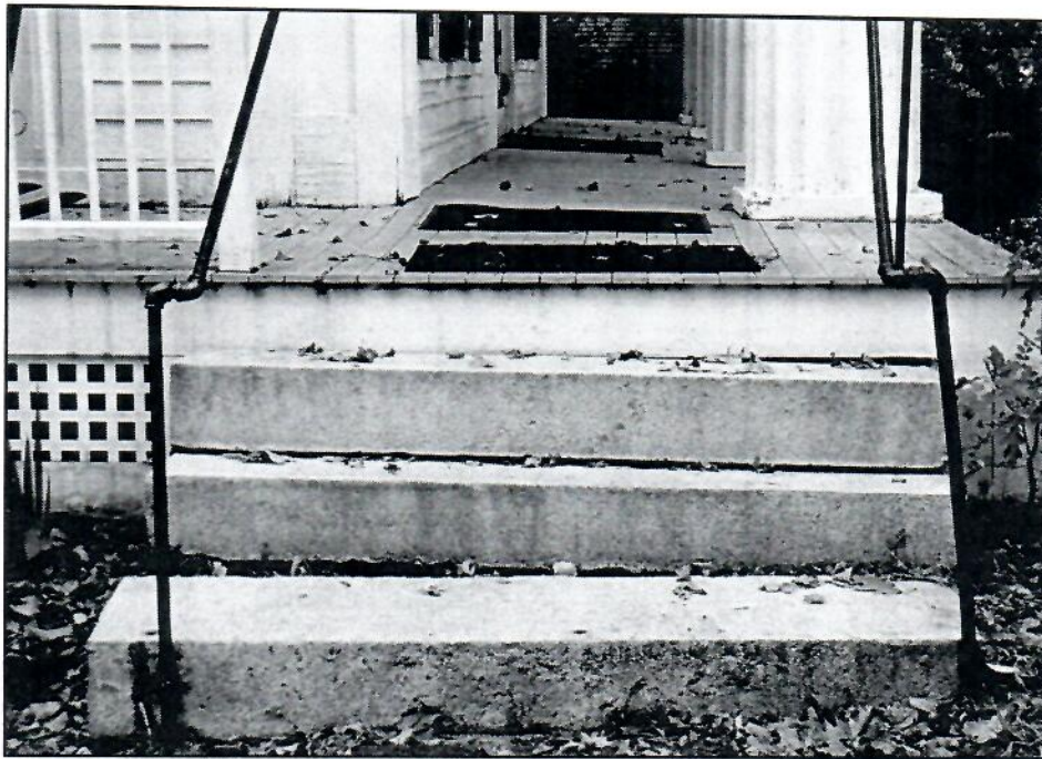
Figure 75: Connection of porch and front portico decks -- stone steps were moved and repositioned to accommodate the transition
