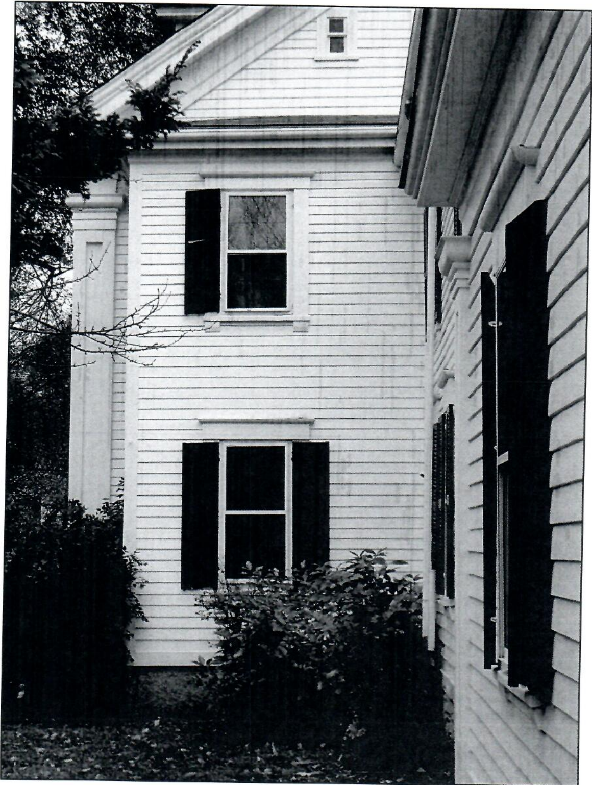
Figure 79: Two-story addition built in two phases against the south wall of main house and its intersection with the west wall of the ell (at right)
