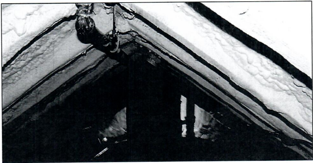
Figure 19: Ell roof rafters, sprayed with insulated foam
