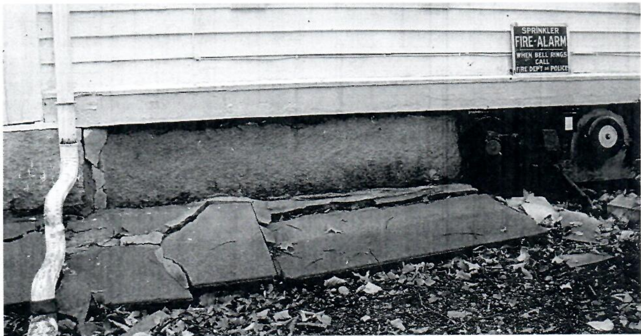
CONCRETE APRON ALONG WEST FOUNDATION WALL TO BE REMOVED
