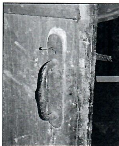
Figure 56: Front and back sides of door to room in NW corner of cellar (top), and original cast iron latch (bottom)
