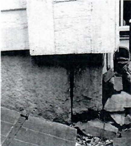
OPEN JOINTS IN FOUNDATION STONES
