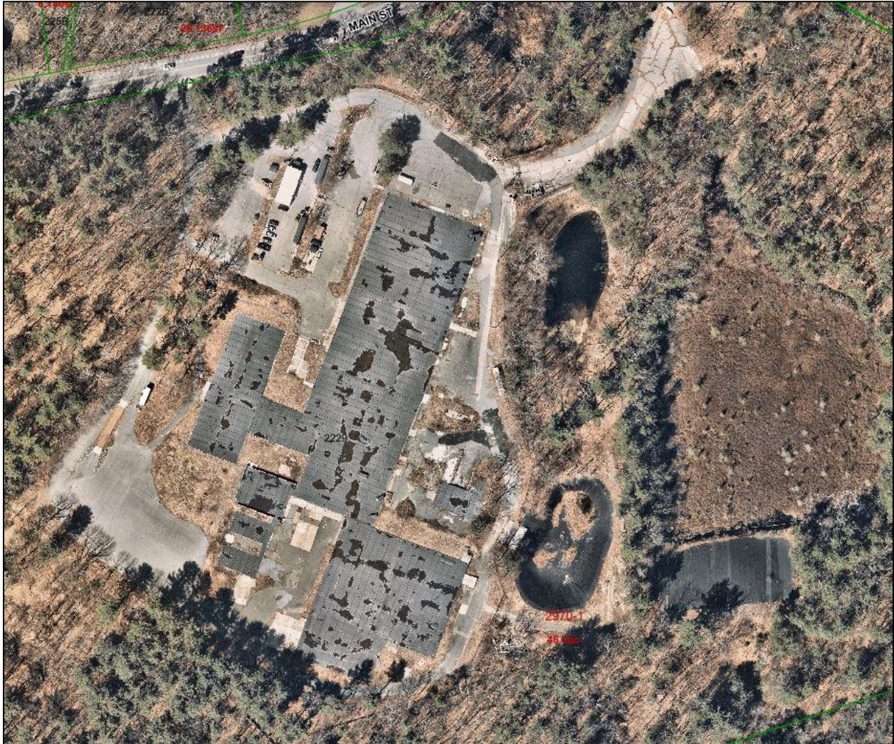
FIGURE 1.3 BUILDING SLABS ADJACENT TO HOLDING BASIN, COOLING WATER RECHARGE POND AND SPHAGNUM BOG
