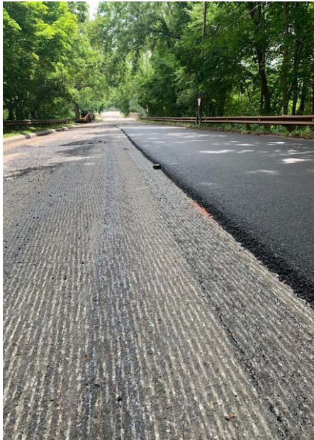
Milling and Filling (Paving)
