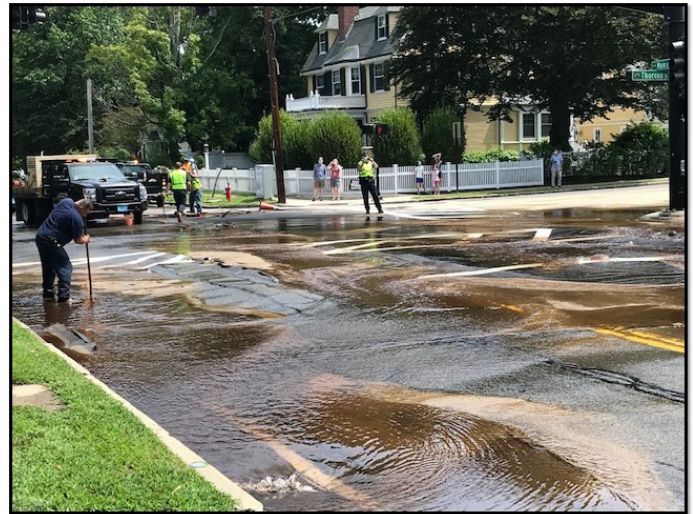
Main and Thoreau Water Main Break
