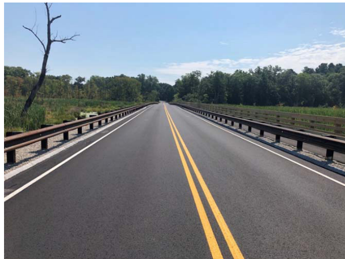
Bridge across Cambridge Turnpike
