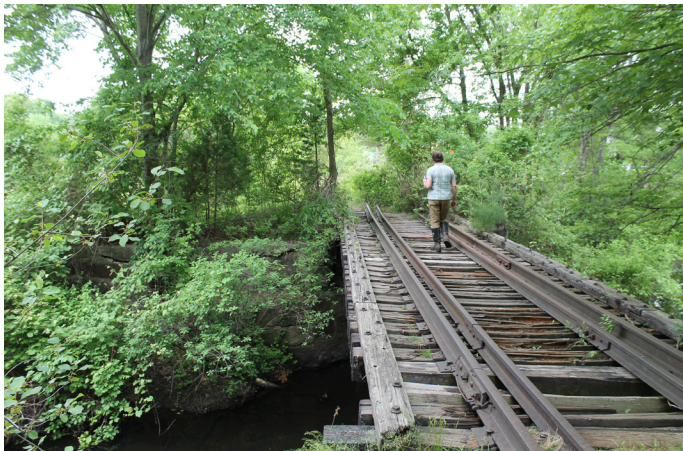
Site walk of the Phase 2B construction on the BFRT
