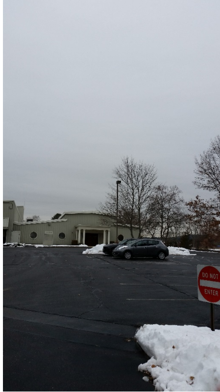
Industrial/Office building on northern side of Winthrop Street
