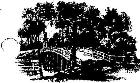
OLD NORTH BRIDGE
