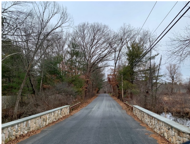
View from bridge, looking toward Carlisle
