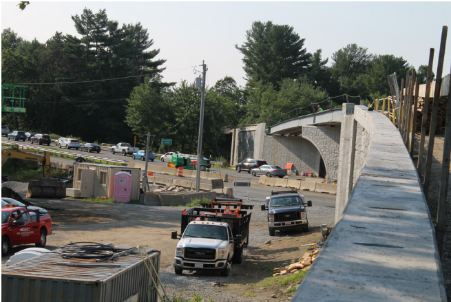
Construction of Phase 2B bridge over Route 2 on the BFRT
