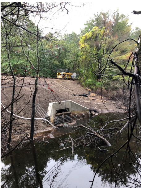
Upstream – Sawmill Brook Culvert Repair
