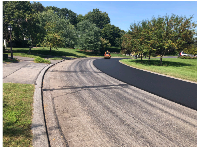
Partridge Lane Final Paving Design, Bidding and Construction of the 2021 Roadway Improvement Project
