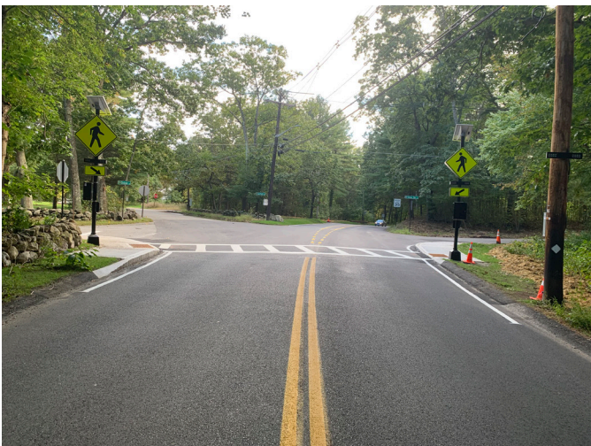
Sudbury Road Crosswalk Completed
