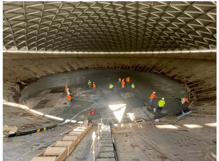
Annursnac Reservoir Improvements Project
