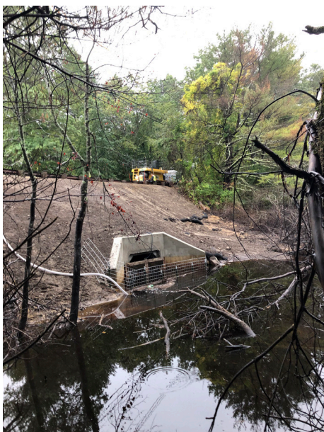
Upstream – Sawmill Brook Culvert Repair
