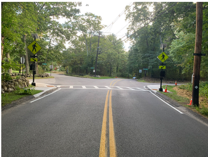
Sudbury Road Crosswalk Completed
