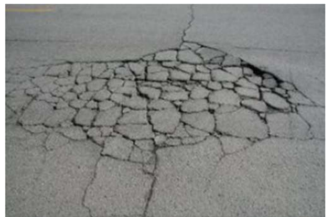
Alligator cracking
