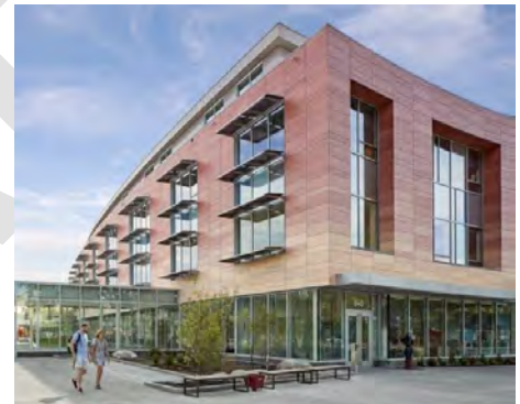
The Cambridge King Open and Cambridge Street Upper School Campus is Net Zero Ready (Photo by Robert Benson) www.mma.org
