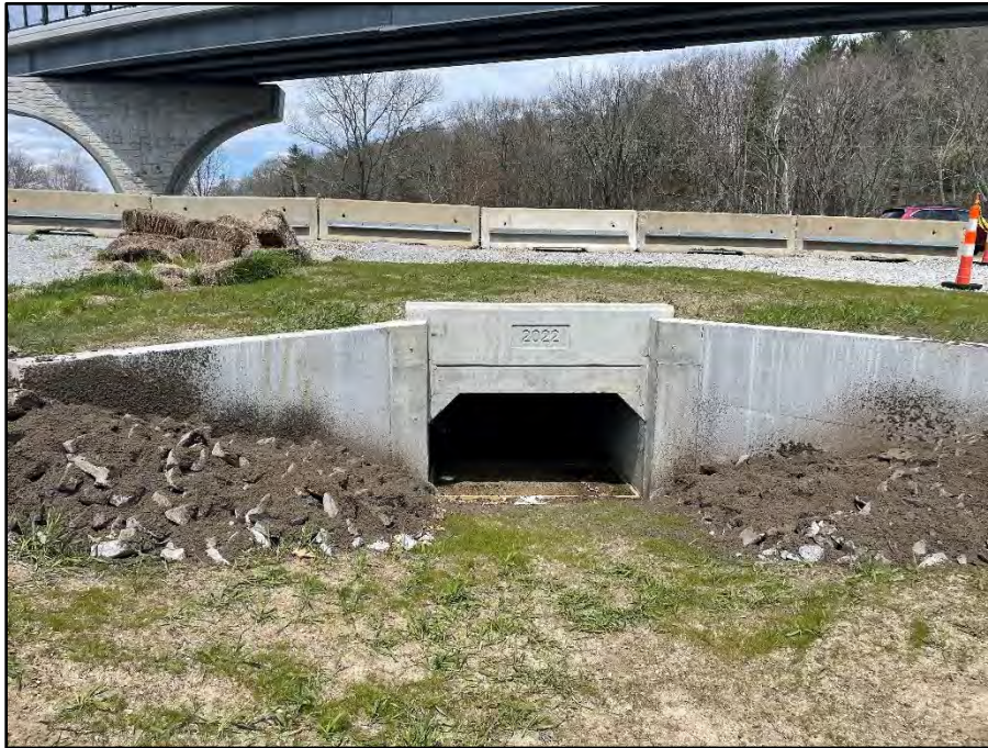
Photo 1. Overview of southern tunnel entrance.
