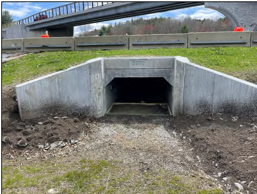
Photo 2. Overview of northern tunnel entrance.
