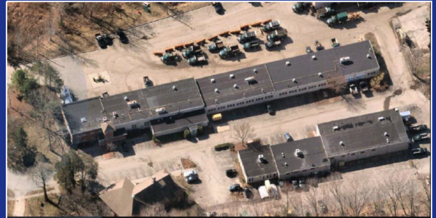
Public Works, Keyes Rd
