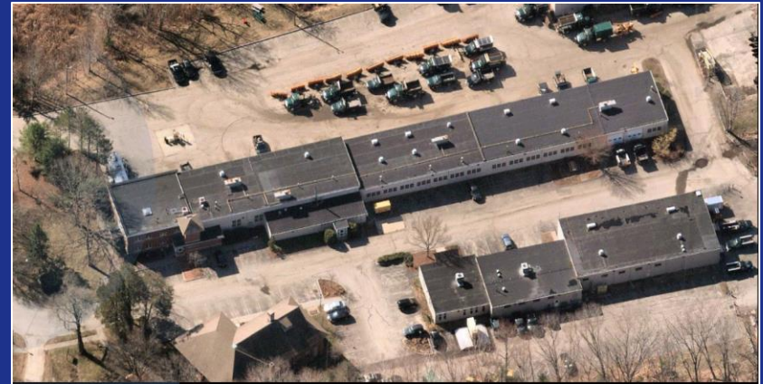
Public Works, Keyes Rd
