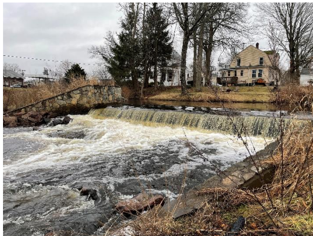
Warner's Pond primary spillway.
