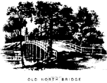
OLD NORTH BRIDGE
