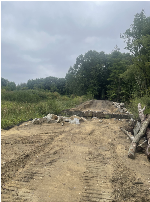
Photo 7: STA 264+00 looking North. Pantry Brook crossing.
