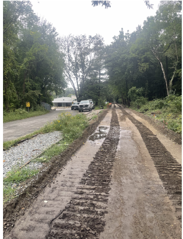
Photo 2: STA 176+00 looking North.
