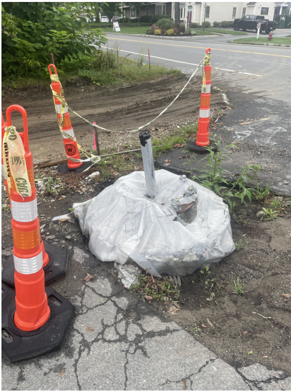
Photo 3: STA 175+50. Signal foundation installed at Ti Sales Driveway is coned off and covered to protect from vehicle damage.
