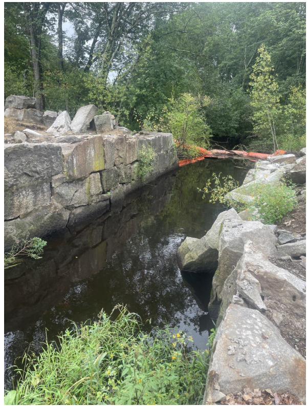
Photo 6: STA 264+50 looking East. Pantry Brook crossing.
