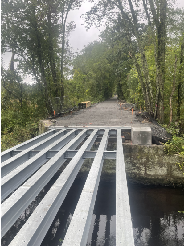
Photo 5: STA 191+00 looking North. Steel Structure at Hop Brook.
