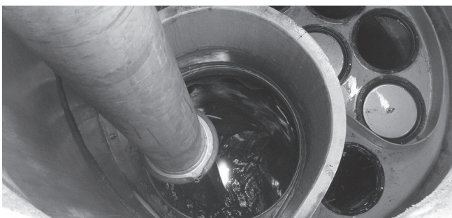
Vacuuming Sump Through MAW
