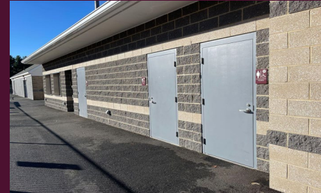
Street Side Concessions and Restrooms
