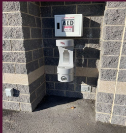
AED machine and bottle filling station
