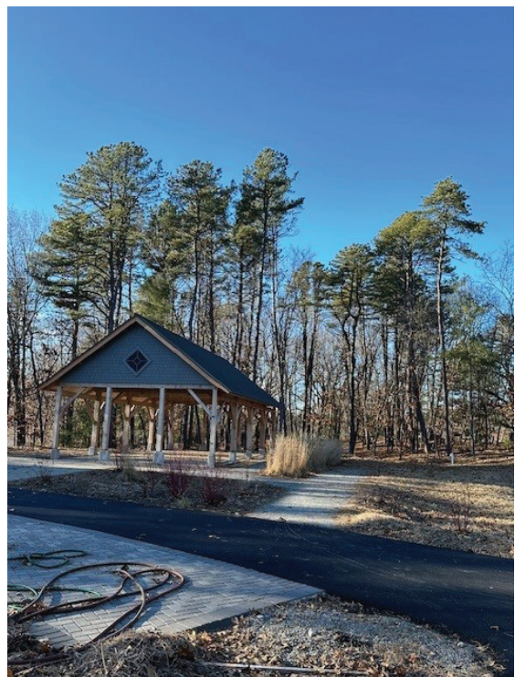
Completed Pavilion Structure
