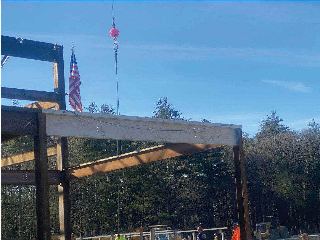
Last steel beam put in place at Topping Off Ceremony
