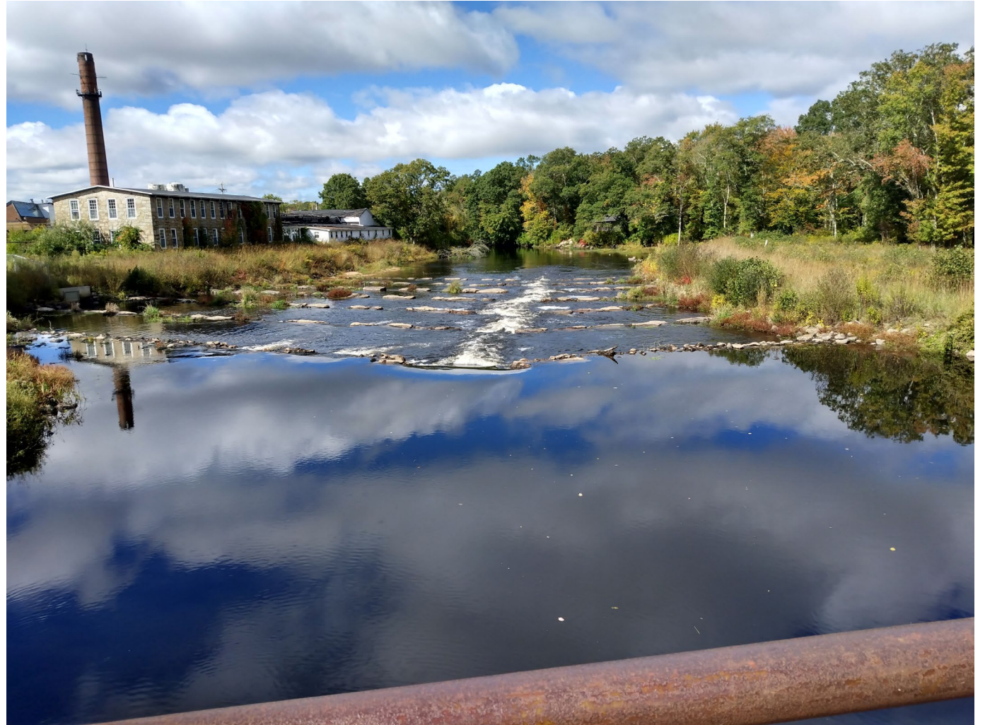
Bradford Dam, Pawcatuck River
