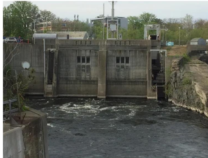
The fish lift at the Essex Dam is just to the left of the former fish ladder, which appears as a concrete ramp. Bjorn Lake/NOAA Fisheries
