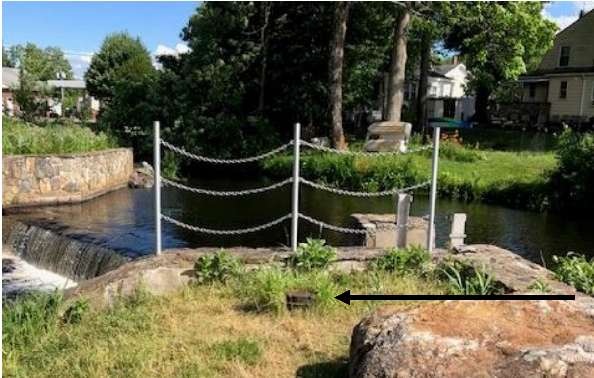
Gate box for valve access
