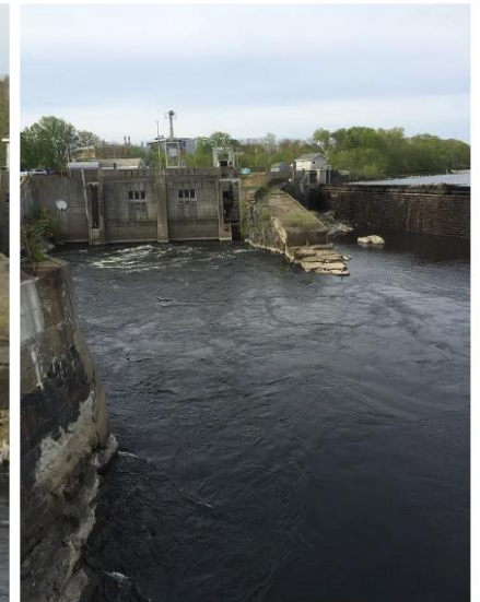
The fish lift at the Essex Dam is just to the left of the former fish ladder, which appears as a concrete ramp. Bjorn Lake/NOAA Fisheries
