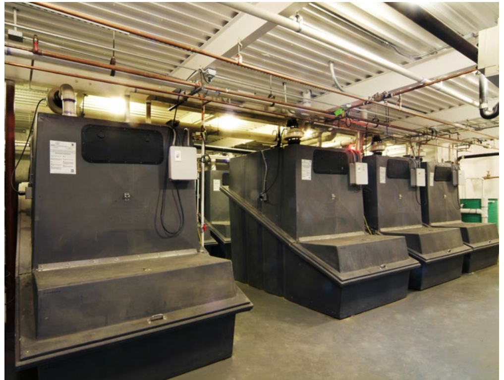
Basement for Composting Tanks
