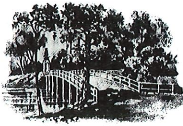
OLD NORTH BRIDGE
