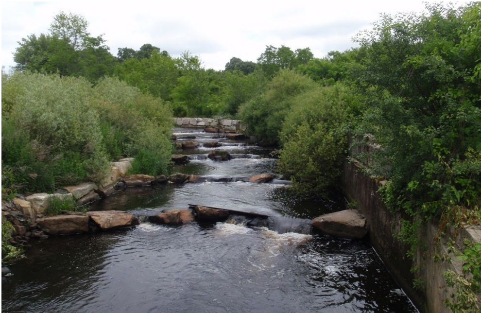
Exhibit 1. Step-pool fishway at the former Sawmill Dam (National Oceanic and Atmospheric Administration [NOAA] 2020)
