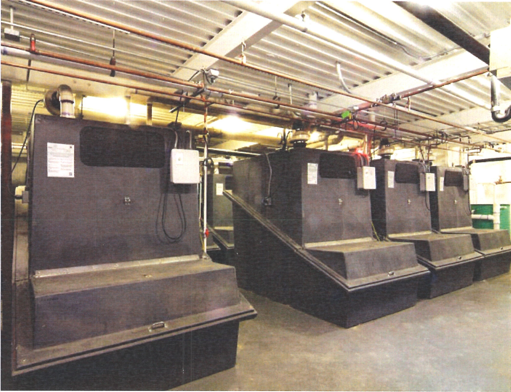
Basement for Composting Tanks
