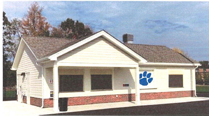
Wood Frame / Siding
