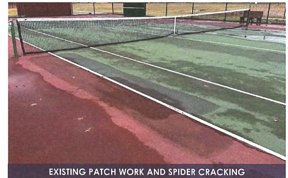
EXISTING PATCH WORK AND SPIDER CRACKING
