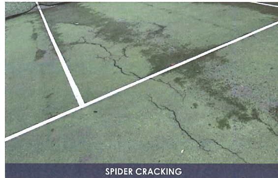
SPIDER CRACKING
