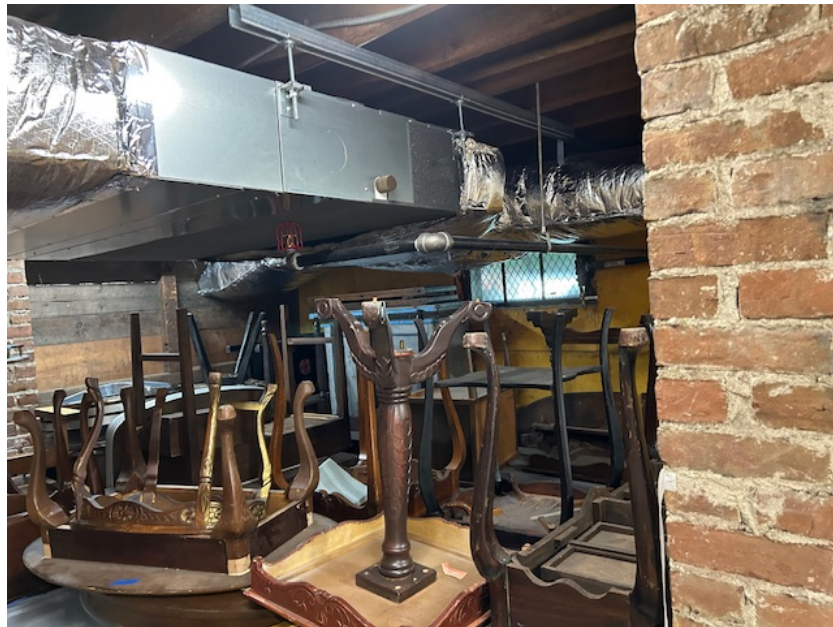
Air handlers and ductwork in the basement
